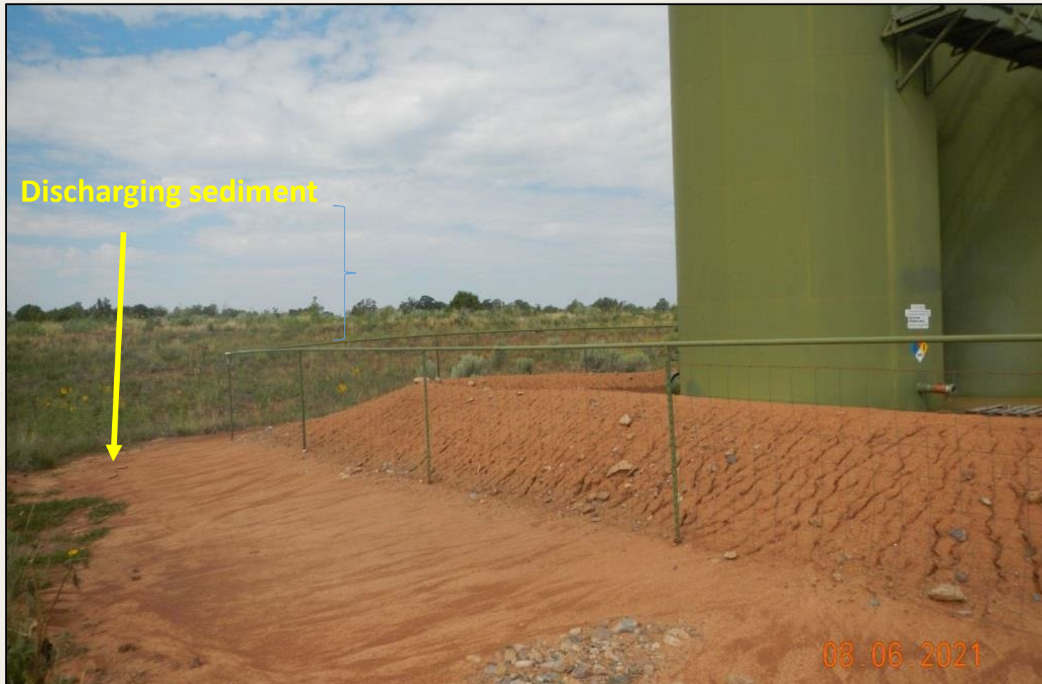
Photo 5. View of sediment discharge and rilling from unstabilized berms around tanks.
