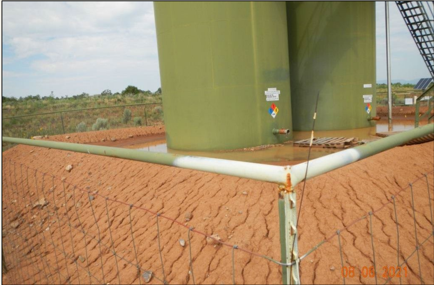
Photo 4. View of eroding berms and water in tank containment. Sediment and water accumulation within containment is resulting in reduced and inadequate containment volume.
