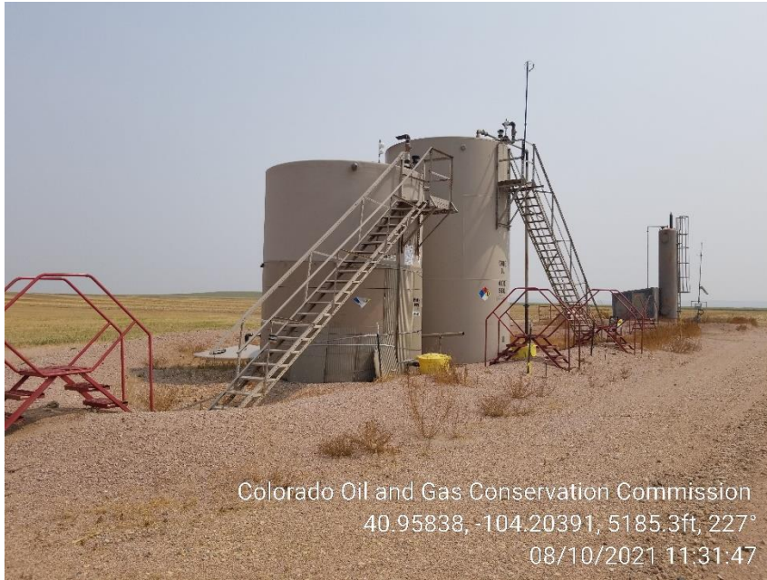
Photo 1 – Tank Battery
