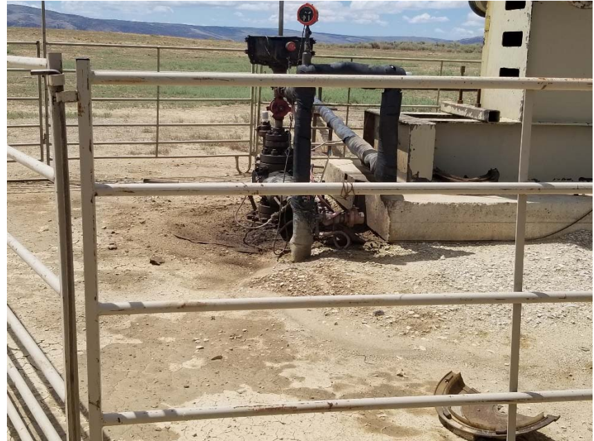
Photo 2. Stained soil at wellhead.
