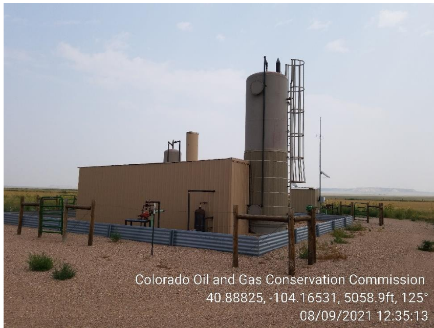
Photo 5 – Heater Treater
