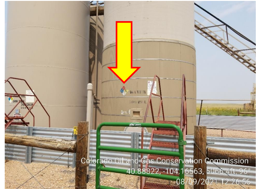
Photo 2 – NFPA Label is Fading. Recommend replacing soon
