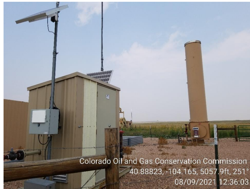
Photo 6 – Gas Meter and ECD
