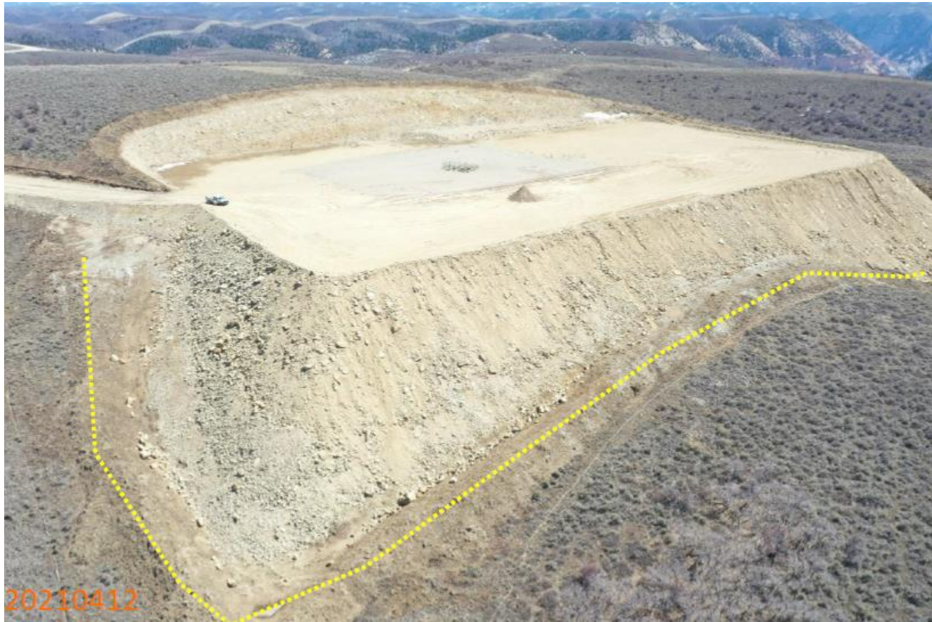
Photo 1: Photos 1-3 used from the 4/12/2021 inspection; photos provide an aerial overview of the Location. Photos show BMPs to protect and stabilize the slopes of the Location are missing or insufficient. It was observed in this inspection that conditions remain unchanged, or have worsened since the 4/12/2021 inspection; erosion degradation evident; large cracks within the fill slope remains; BMPs to address stabilization concerns remain missing.
