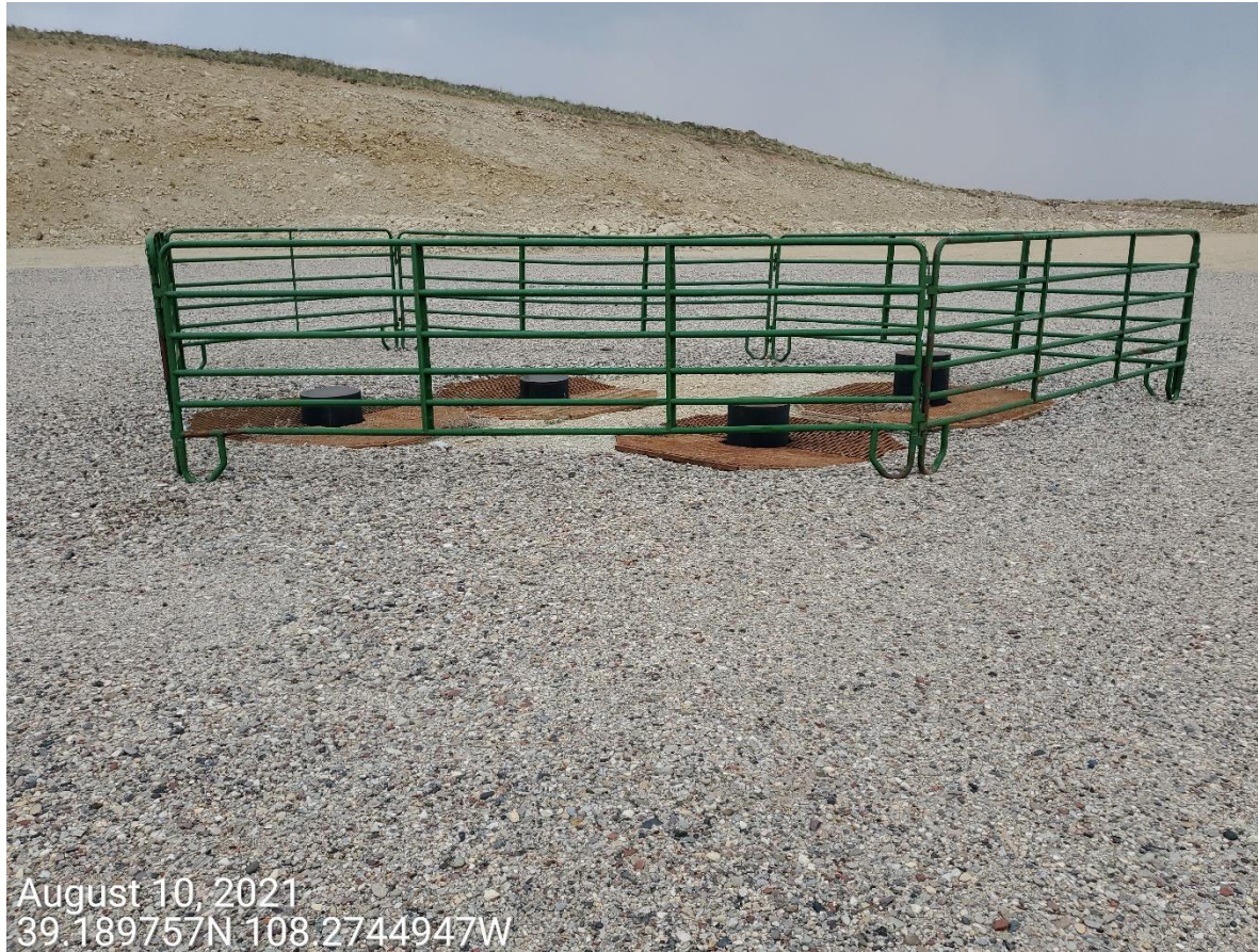
Photo 8: Photo shows 4 conductors remain on the location; no drilling operations have commenced.
