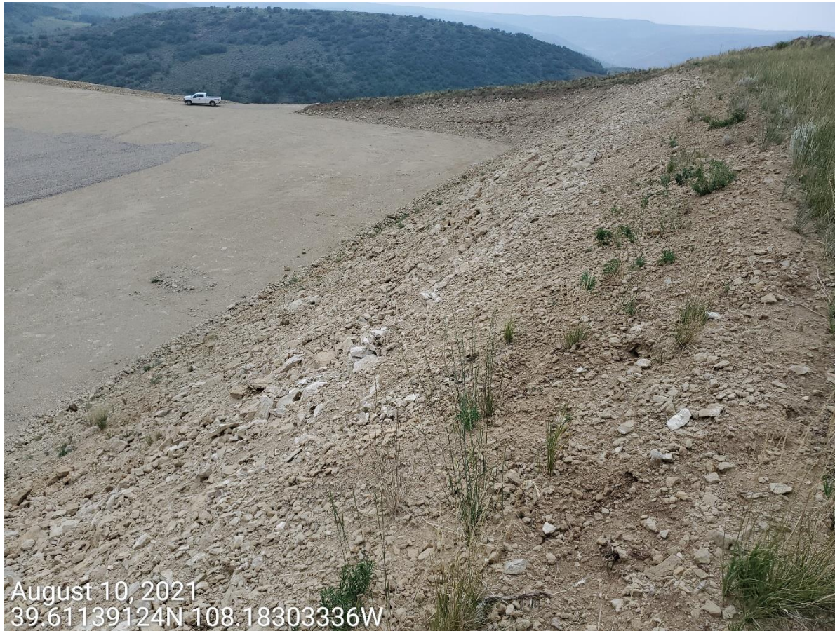
Photo 5: Photo taken from the cut slopes of the Location. Photos show BMPs to protect and stabilize slopes of the Location remain missing or insufficient.
