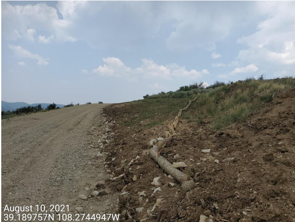
Photo 6: Photo taken from the access road. Photo shows cut slopes of the access road have been regraded; areas reclaimed and hydromulch applied.
