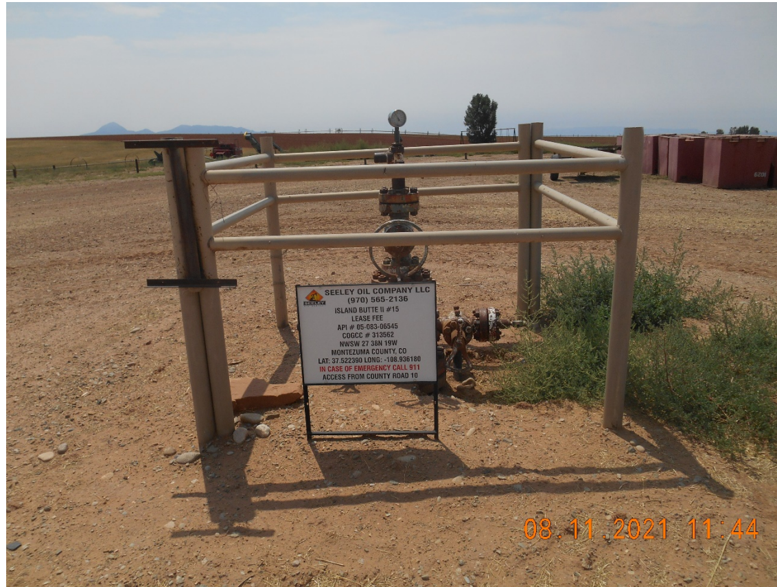
Injection Wellhead – Temporarily Abandoned
