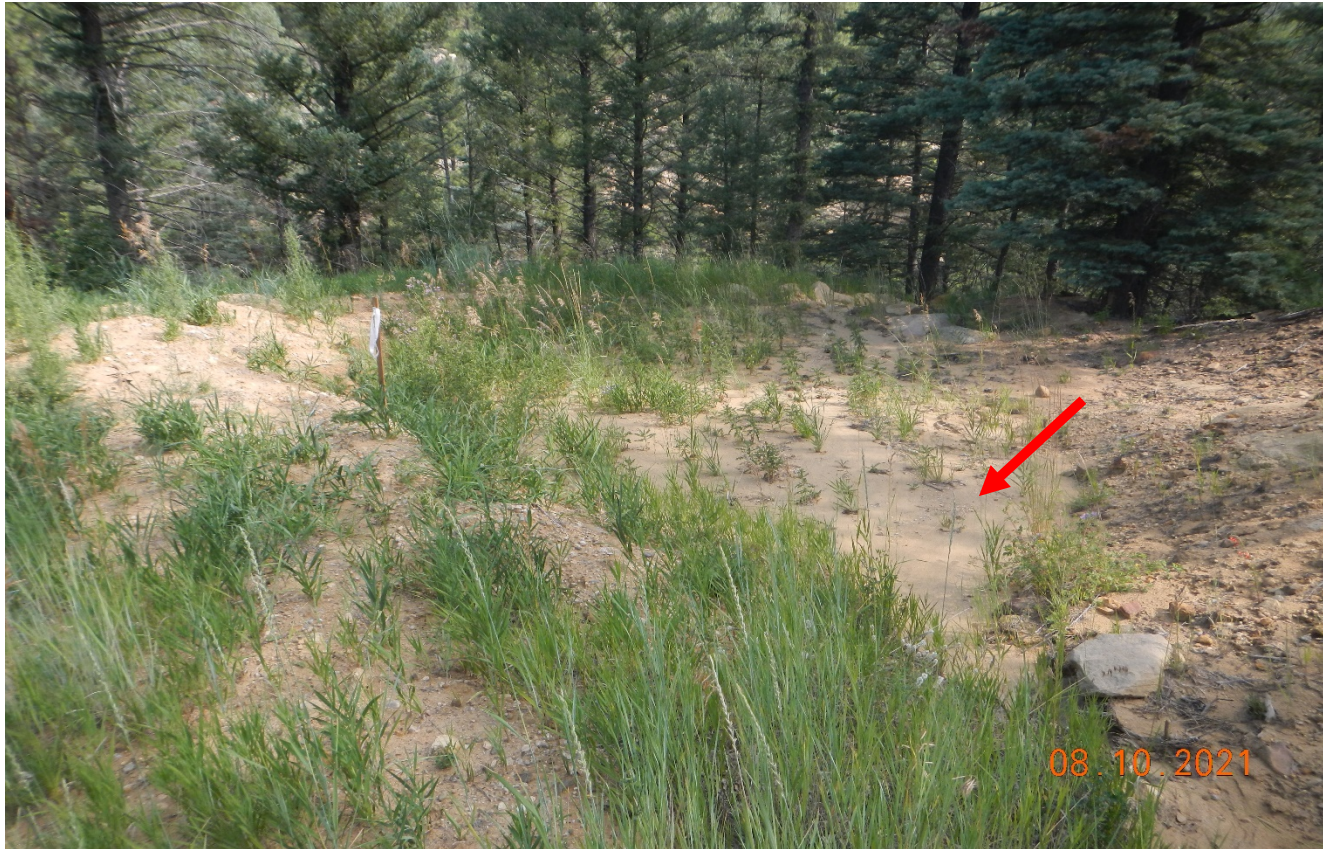
Photo 3. There is a sediment trap along the access road that is filled in with sediment. The sediment trap was not cleaned out. This could have been done by hand to avoid vegetation disturbance at the area shown at red arrow. Previous correction action was not performed.
