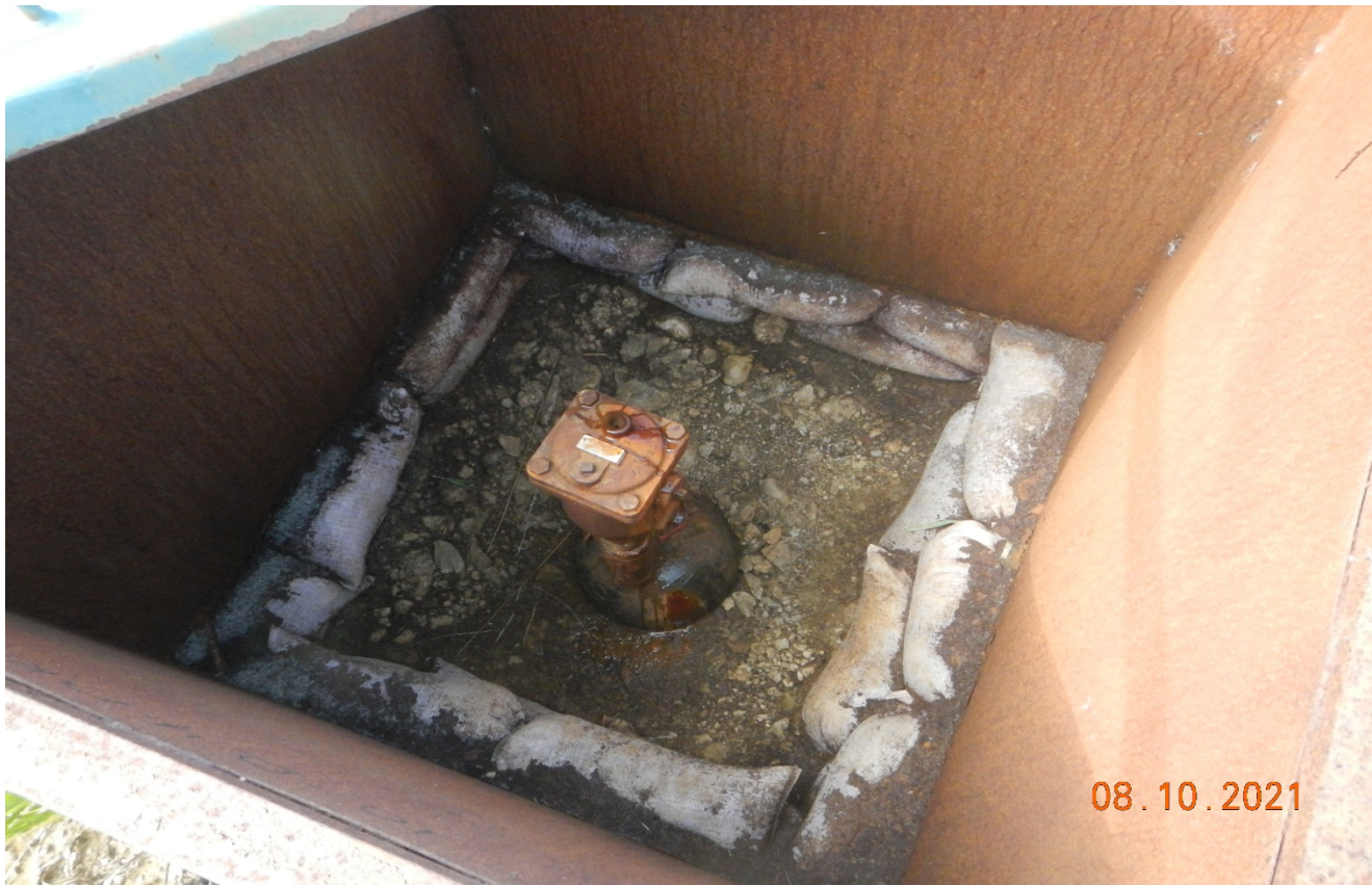
Photo 5. There was a slight PW drip at the valve inside the box.
