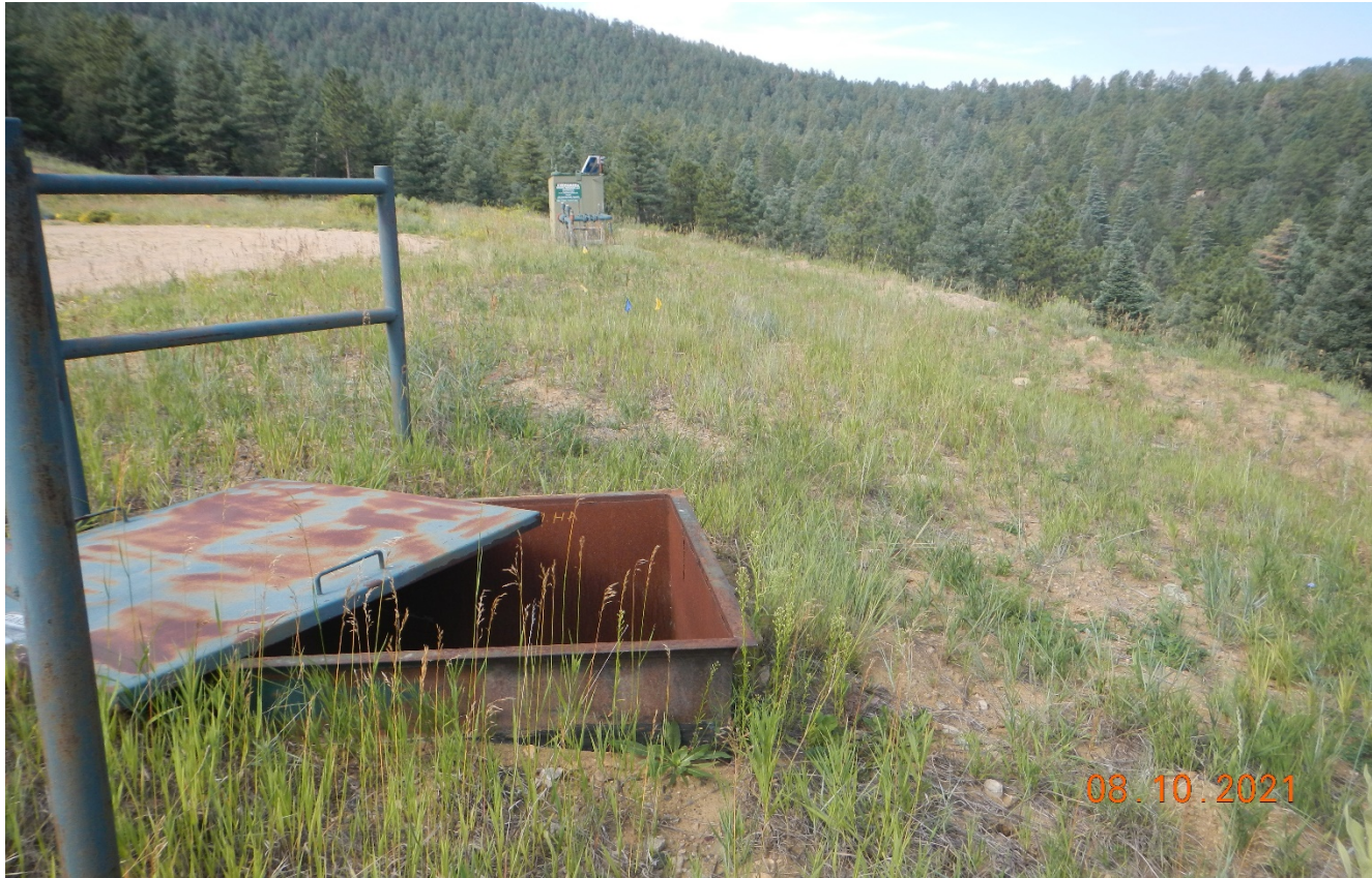
Photo 4. Facing west toward the location fill slope. The valve box lid was left open and needs to be kept closed to prevent entry.
