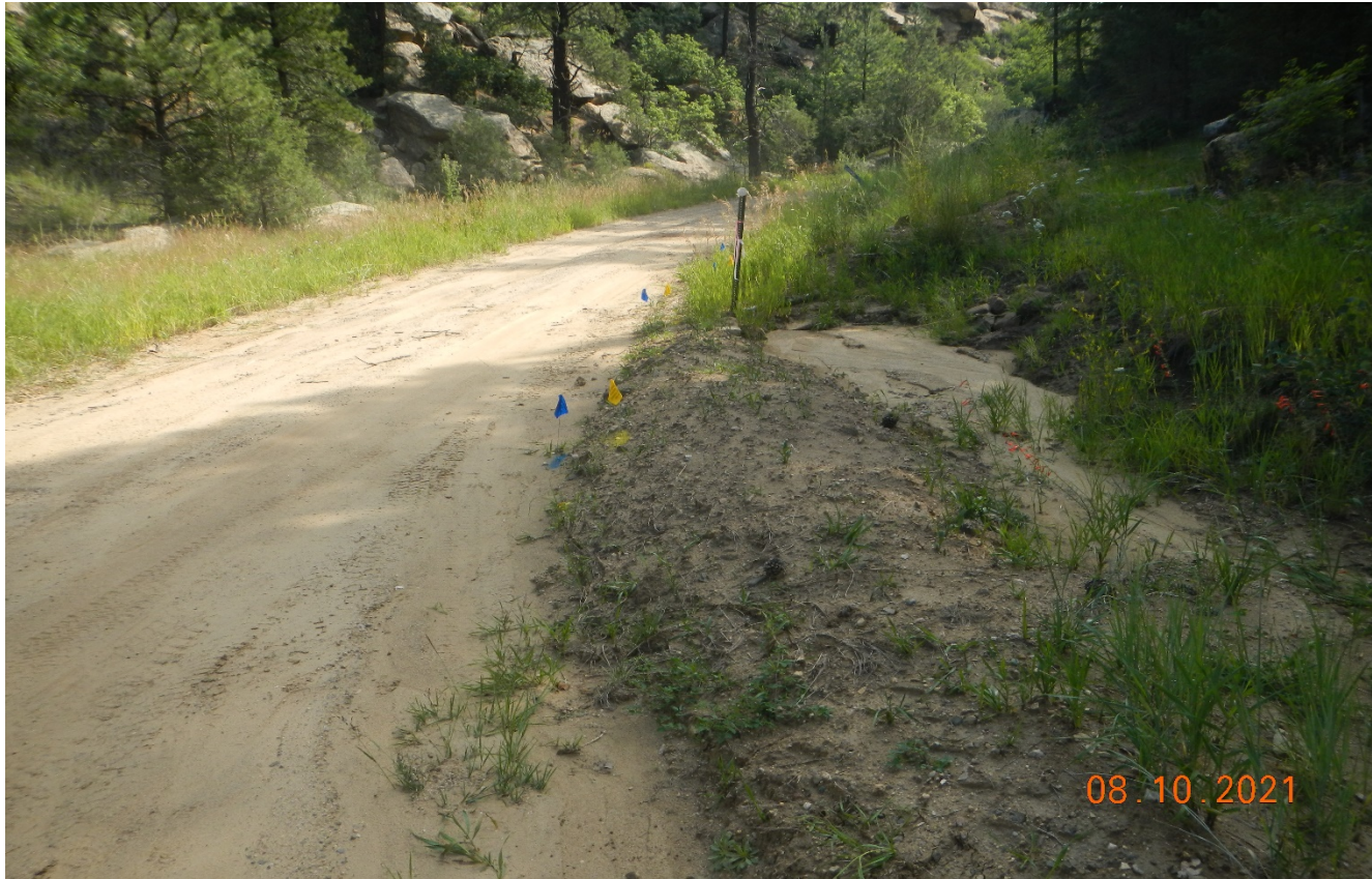
Photo 1. There is culvert at the beginning of the access road in the canyon that is filled in with sediment.
