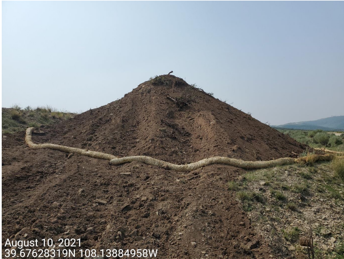
Photo 4: Photo shows example of stockpiled soils with a erosion log installed at base; BMPs to stabilize and protect soils currently missing.
