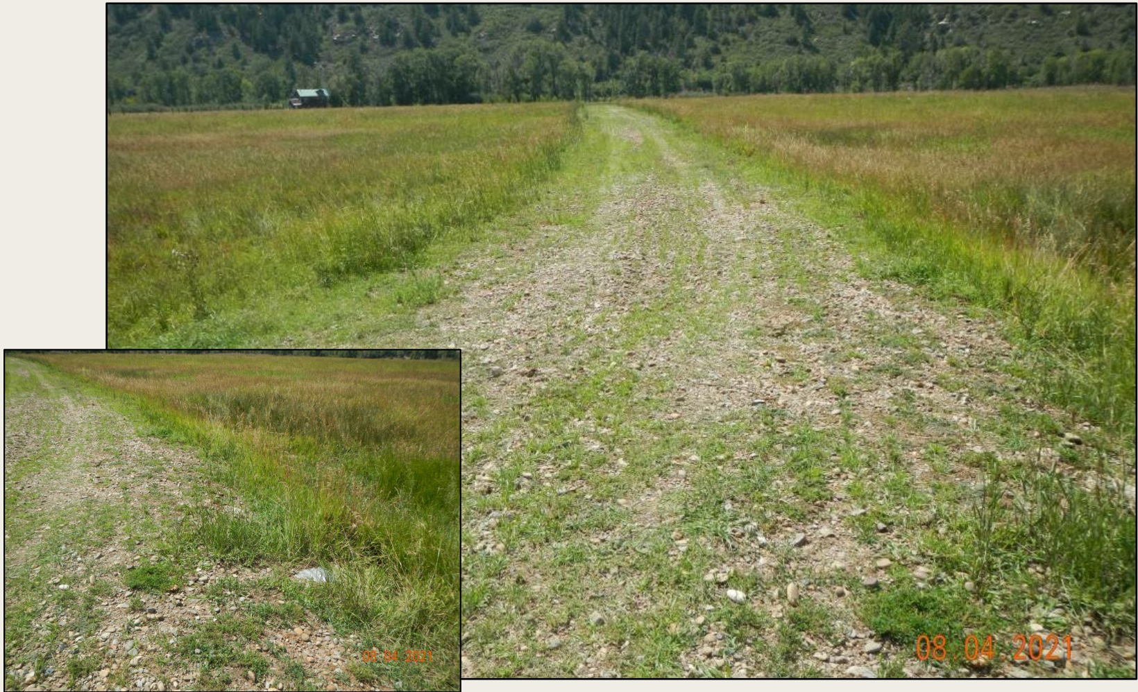
Photo 1. View of the access road from the access entrance facing north toward the well pad. Road fill, gravel, and culvert (inset) remain in place.
