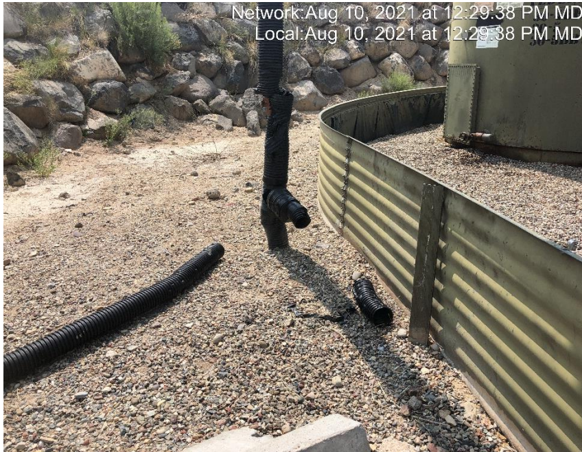
Photo #4740 Flow line heating insulation open ended and not capped.
