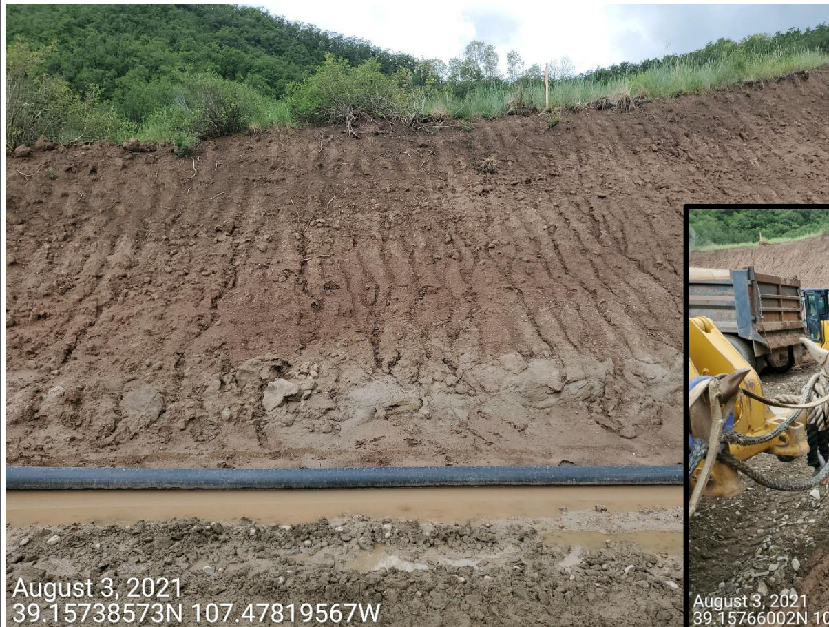
Photo 4: Photo taken from the cut slopes on the east end of the Location. Photo shows stormwater and erosion control measures to protect/stabilize the slopes of the Location remain missing or inadequate.
