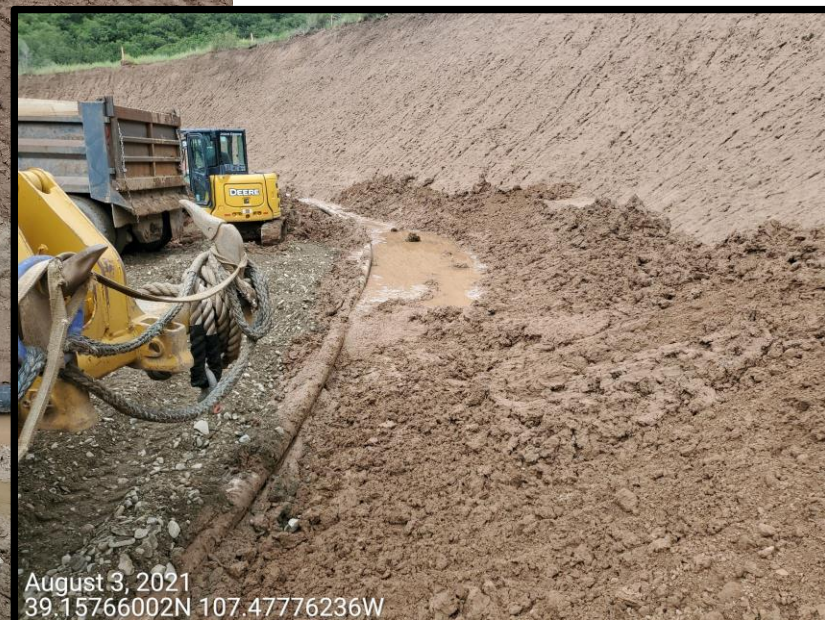
Photo 4: Photo taken from the cut slopes on the east end of the Location. Photo shows stormwater and erosion control measures to protect/stabilize the slopes of the Location remain missing or inadequate.
