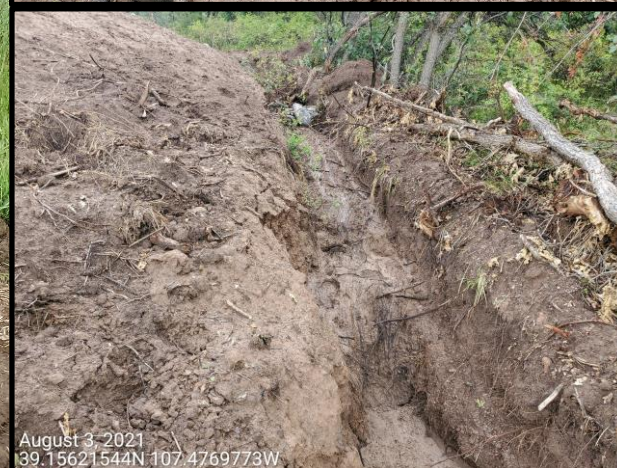
Photo 10: Photo taken from the stormwater “ditch” leading from the Location. Photos show BMPs remain improperly constructed with vertical slopes and extracted soils left along channel remain unconsolidated and a pollutant source .
