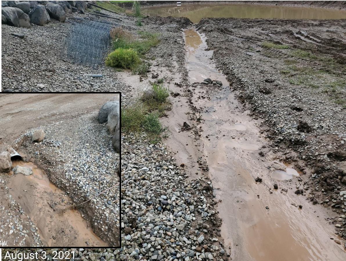
Photo 11: Photo shows stormwater and sediment discharge from the Location has filled the stormwater ditches and culvert.
