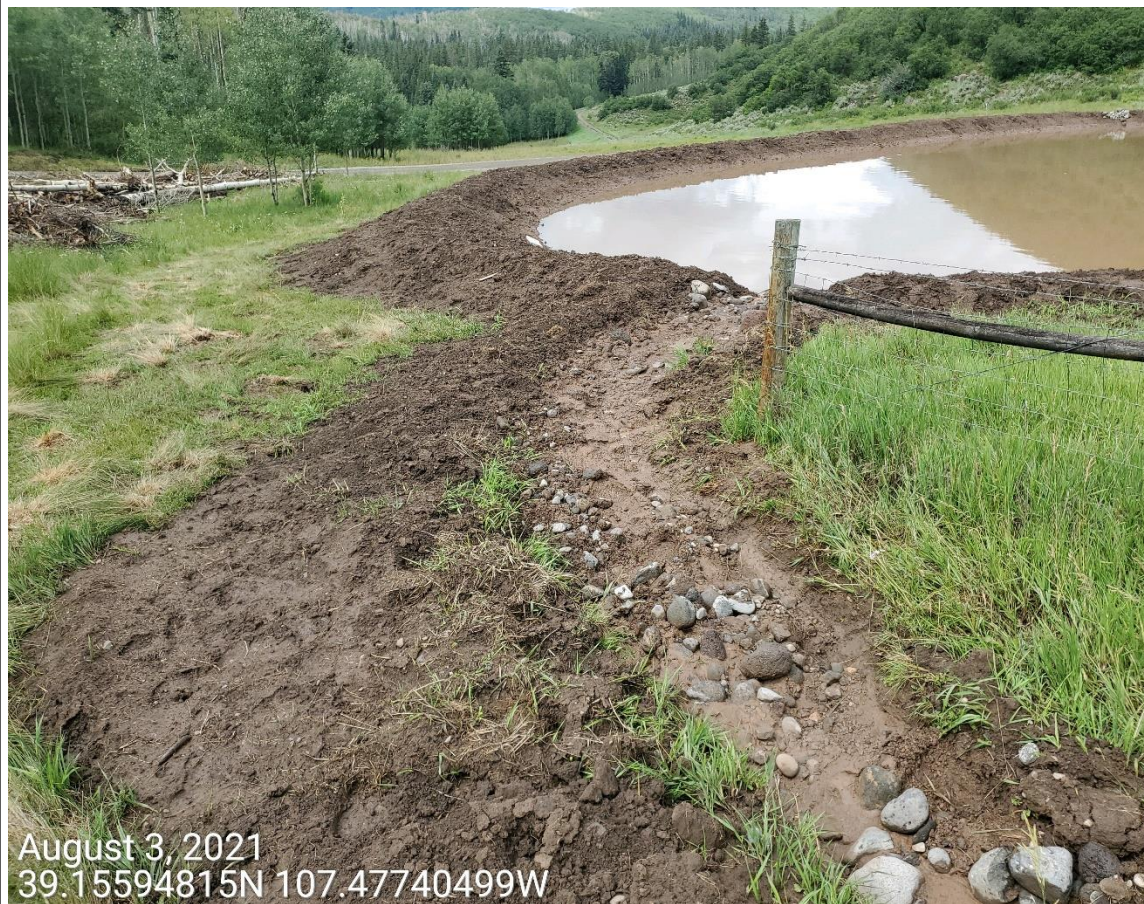
Photo 12: Photo taken from the sediment trap/pond west of the Location. Previous inspection documented that the inlets were inadequate. Photos show inlets remain inadequate.
