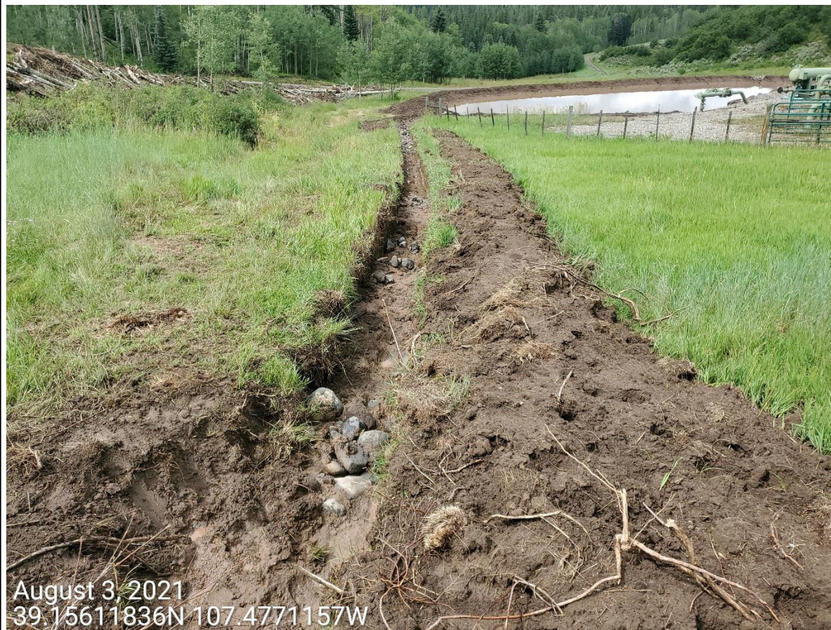
Photo 10: Photo taken from the stormwater “ditch” leading from the Location. Photos show BMPs remain improperly constructed with vertical slopes and extracted soils left along channel remain unconsolidated and a pollutant source .
