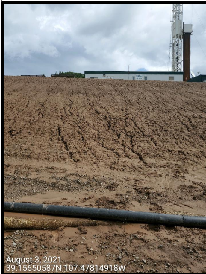
Photo 2: Photo taken from the fill slopes on the west end of the Location. Photo shows stormwater and erosion control measures to protect/stabilize the slopes of the Location, and to properly manage discharge remains missing or inadequate.
