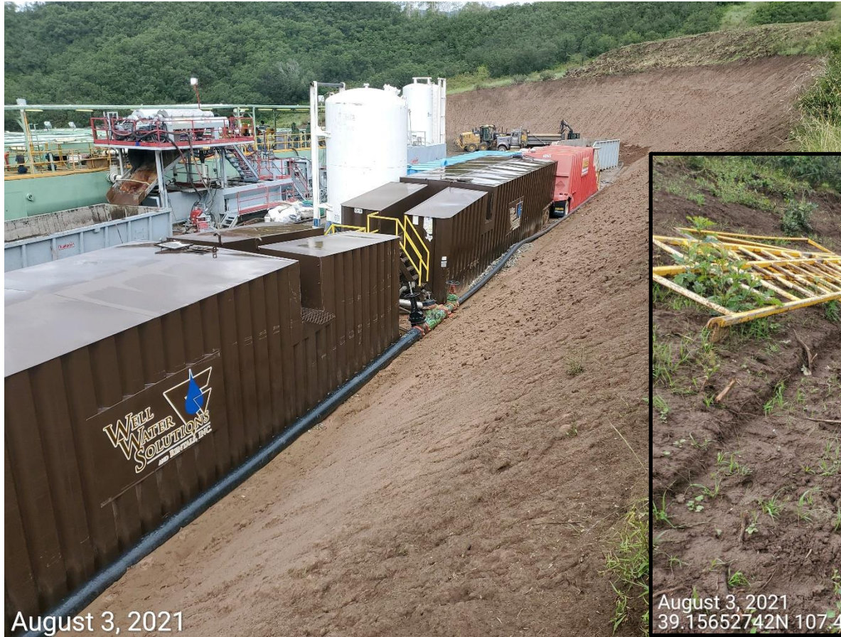
Photo 8: Photo shows equipment remains improperly stored/placed within the stormwater diversion ditch on the eastern and southern perimeter of the pad.
