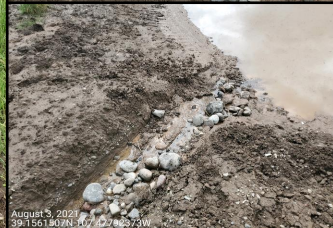
Photo 12: Photo taken from the sediment trap/pond west of the Location. Previous inspection documented that the inlets were inadequate. Photos show inlets remain inadequate.
