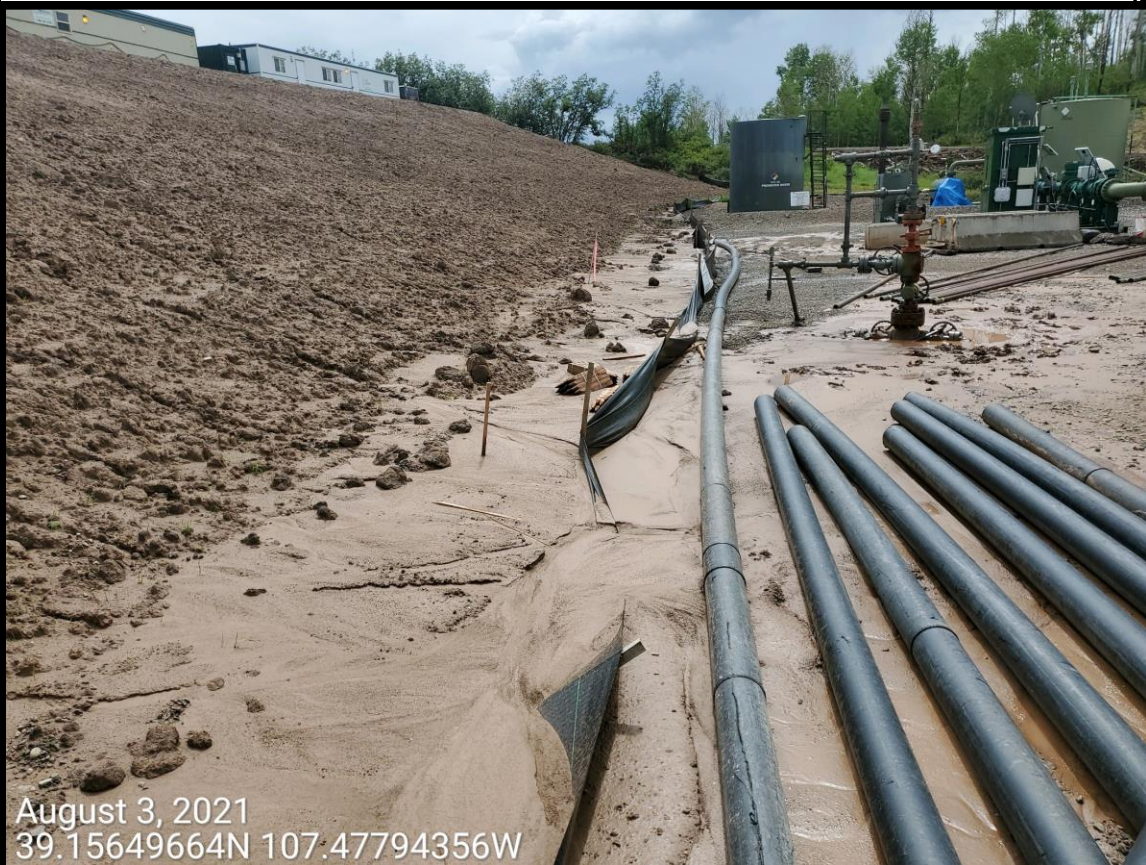
Photo 2: Photo taken from the fill slopes on the west end of the Location. Photo shows stormwater and erosion control measures to protect/stabilize the slopes of the Location, and to properly manage discharge remains missing or inadequate.
