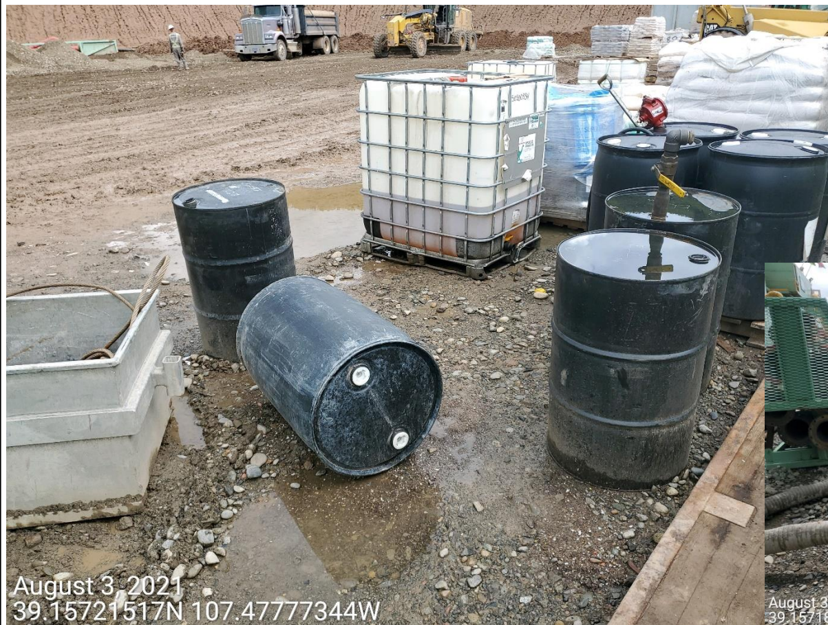
Photo 16: Photo shows example of barrels/tanks/containers observed stored on the Location without proper secondary containment. This issue was documented in the previous inspection; BMPs remain missing or insufficient to contain a spill.
