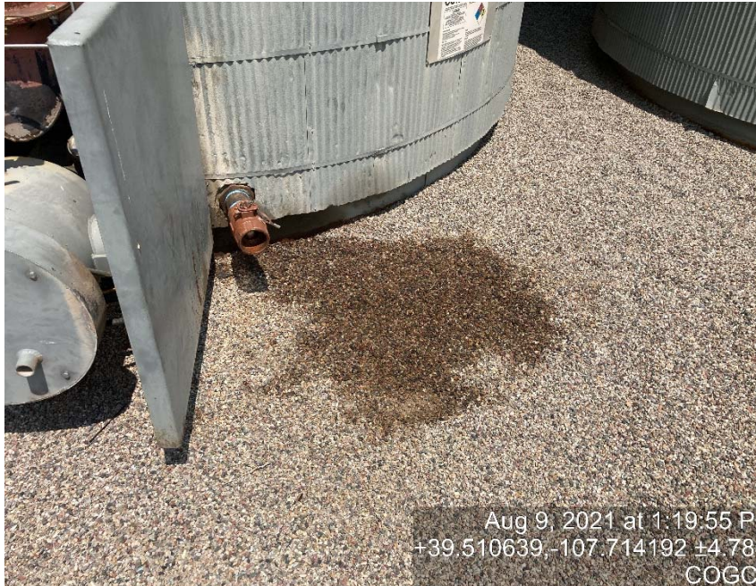
Lack of bull plug/staining
