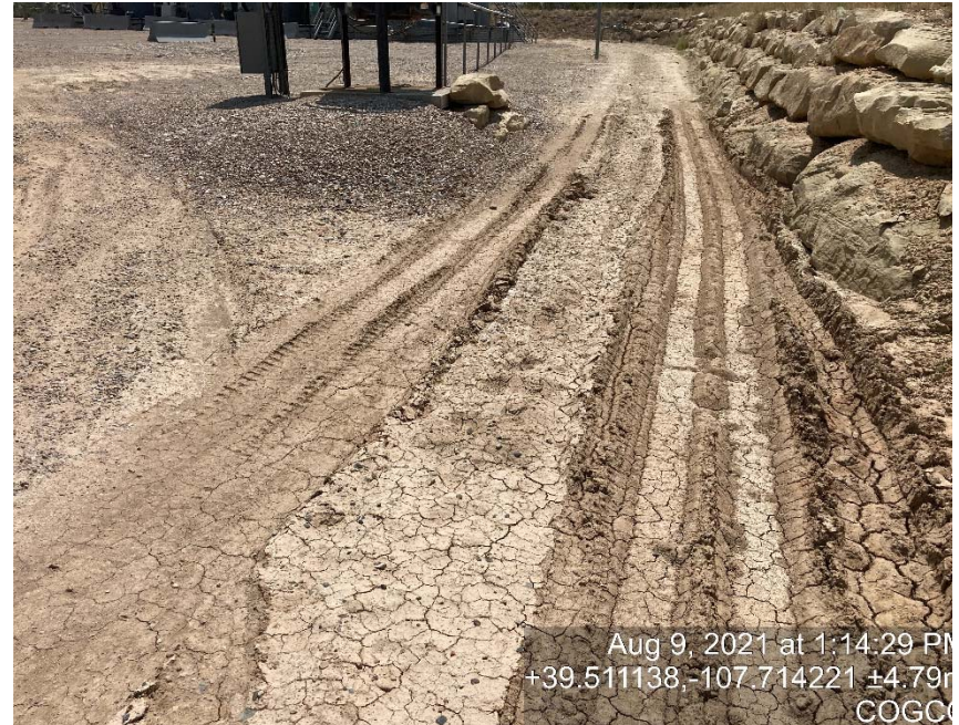
Lack of stabilization/compaction
