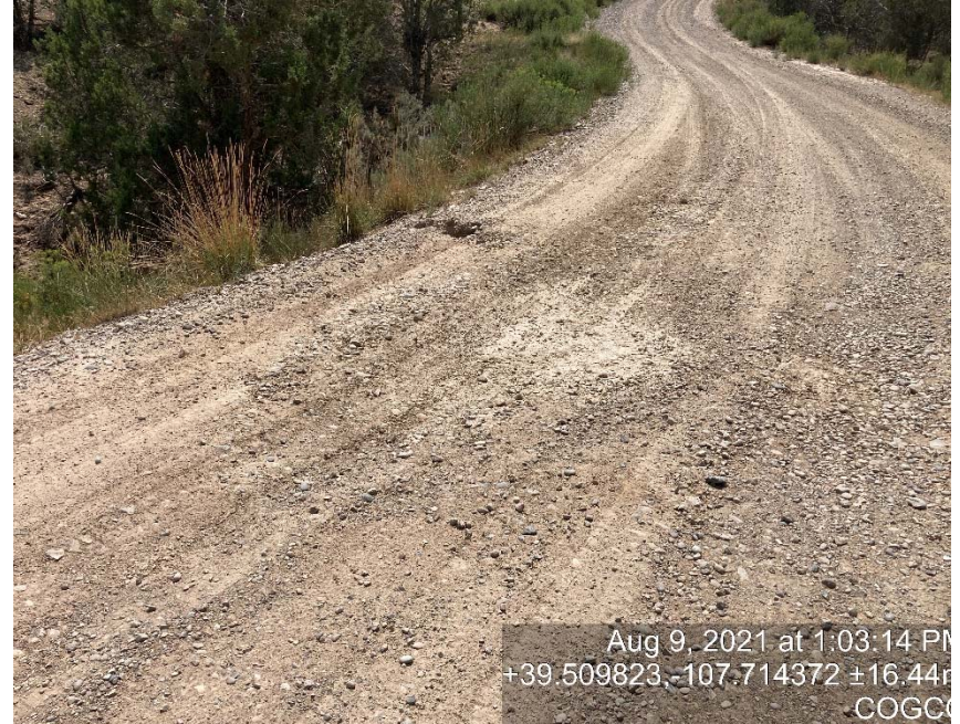
Lack of stabilization/ erosion on access road
