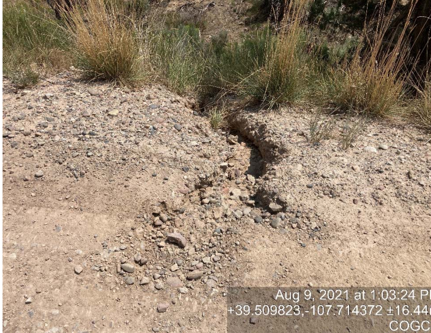
Lack of stabilization/ erosion on access road
