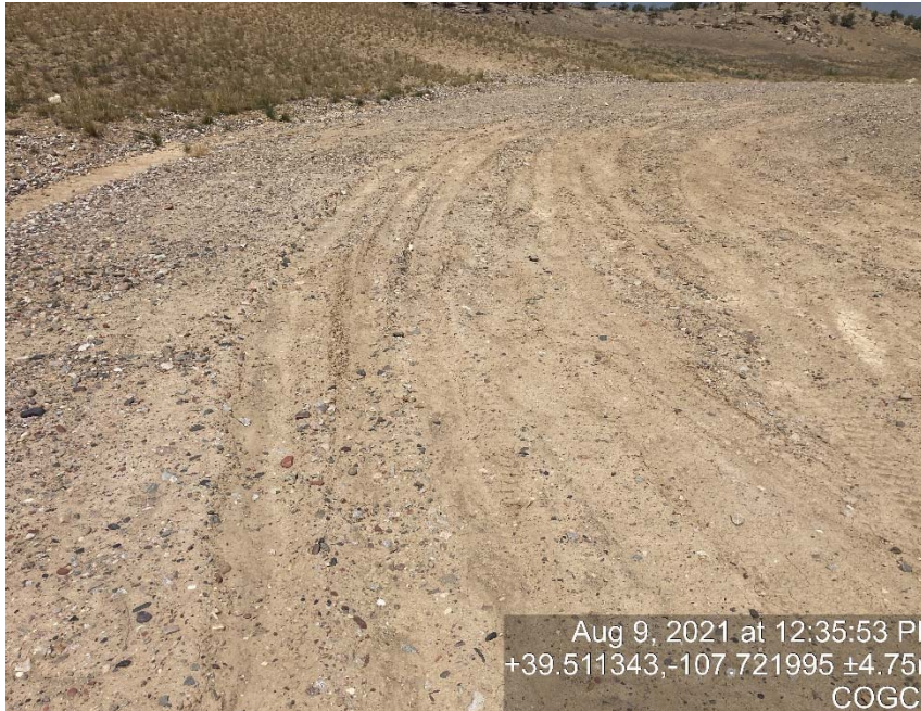
Lack of stabilization/compaction
