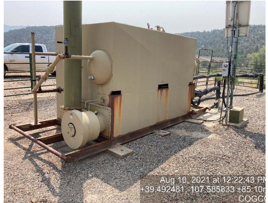
location/lack of labeling of contents in bath
