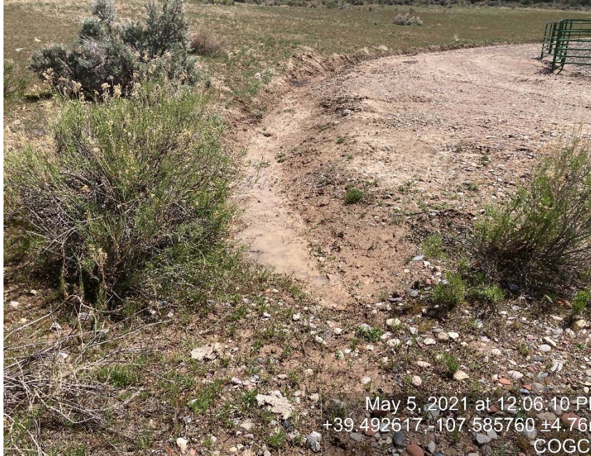
Previous inspection photo of ditch around location
