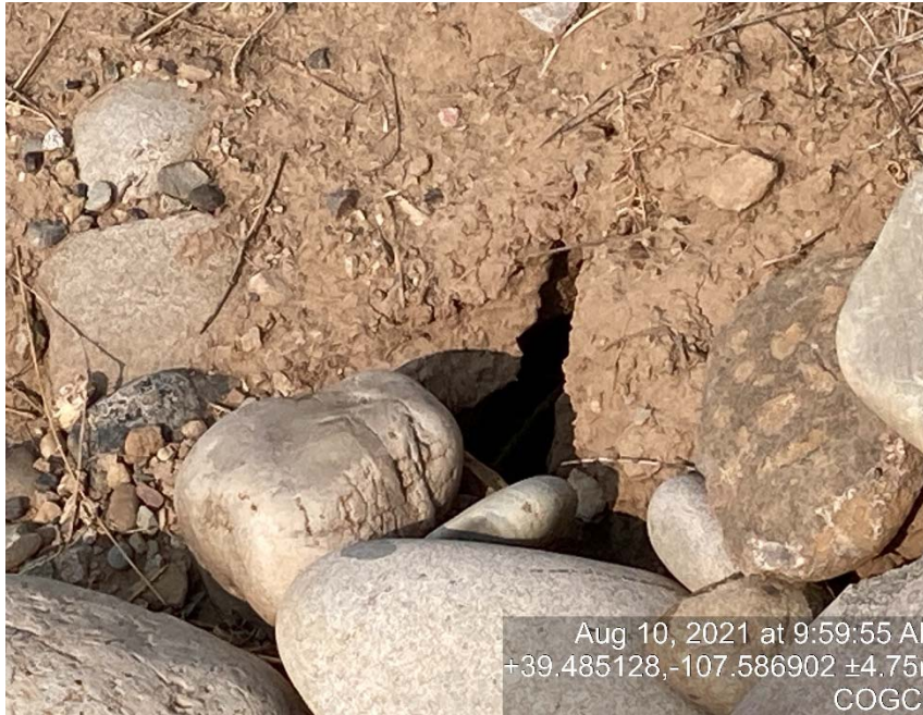
Sediment trap undermining
