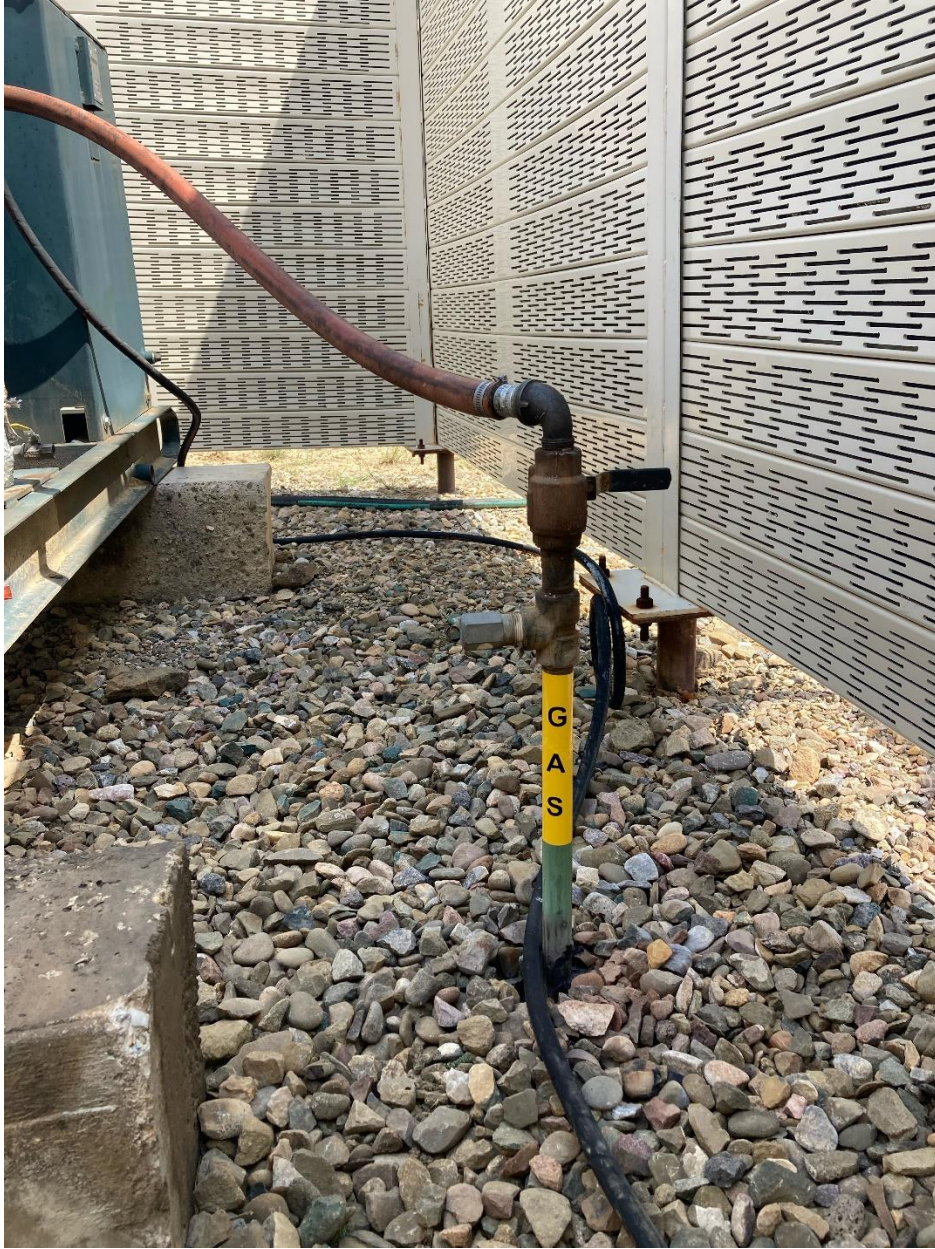
Marked riser to comply with Rule 603.f.
