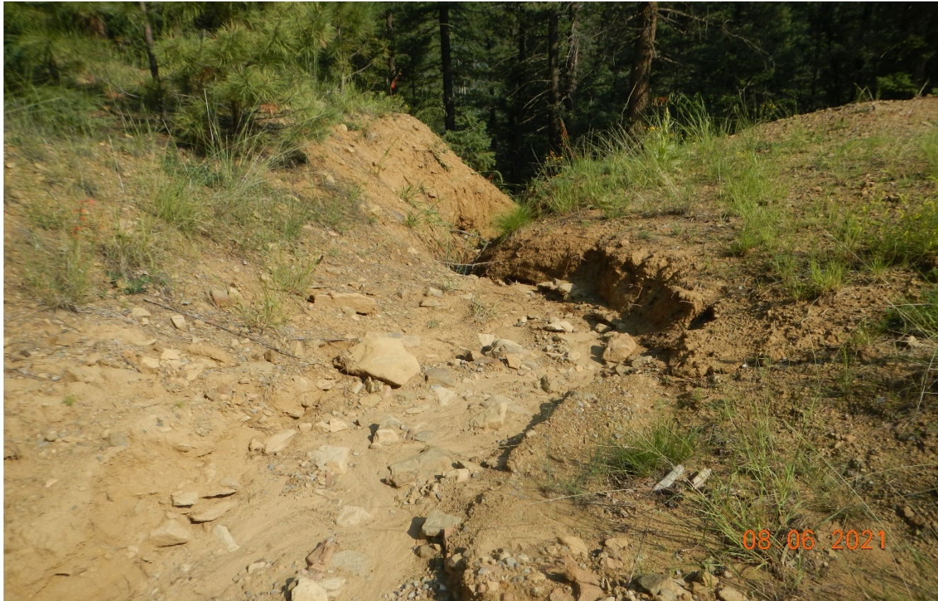
Photo 5. The erosion gully at the second switchback of the road was not repaired/stabilized.
