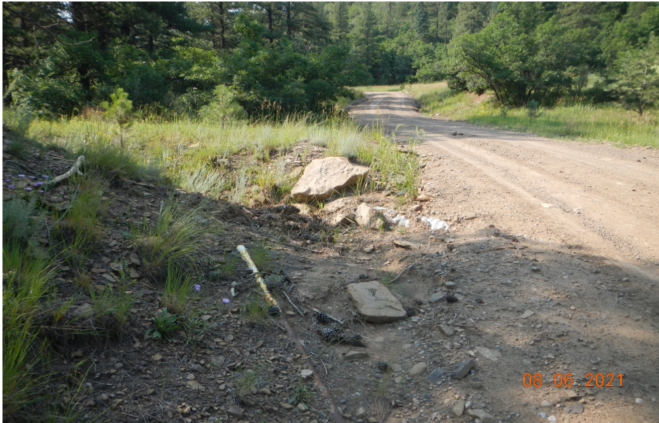
Photo 2. There is metal pipe markers laying on the ground near the culverts. The pipe needs to be removed or reinstalled.
