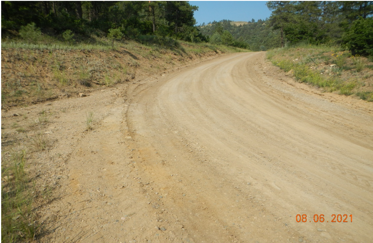
Photo 4. Facing west at the switch back of the road where there was vehicle rutting. The road was graded however, the road was not stabilized and vehicle rutting may occur during wet winter condition.
