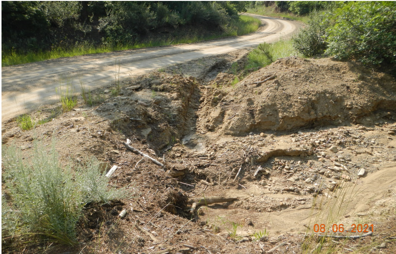
Photo 3. It appears this culvert was cleaned out in the canyon and has since filled back in with debris. Ongoing maintenance is required.
