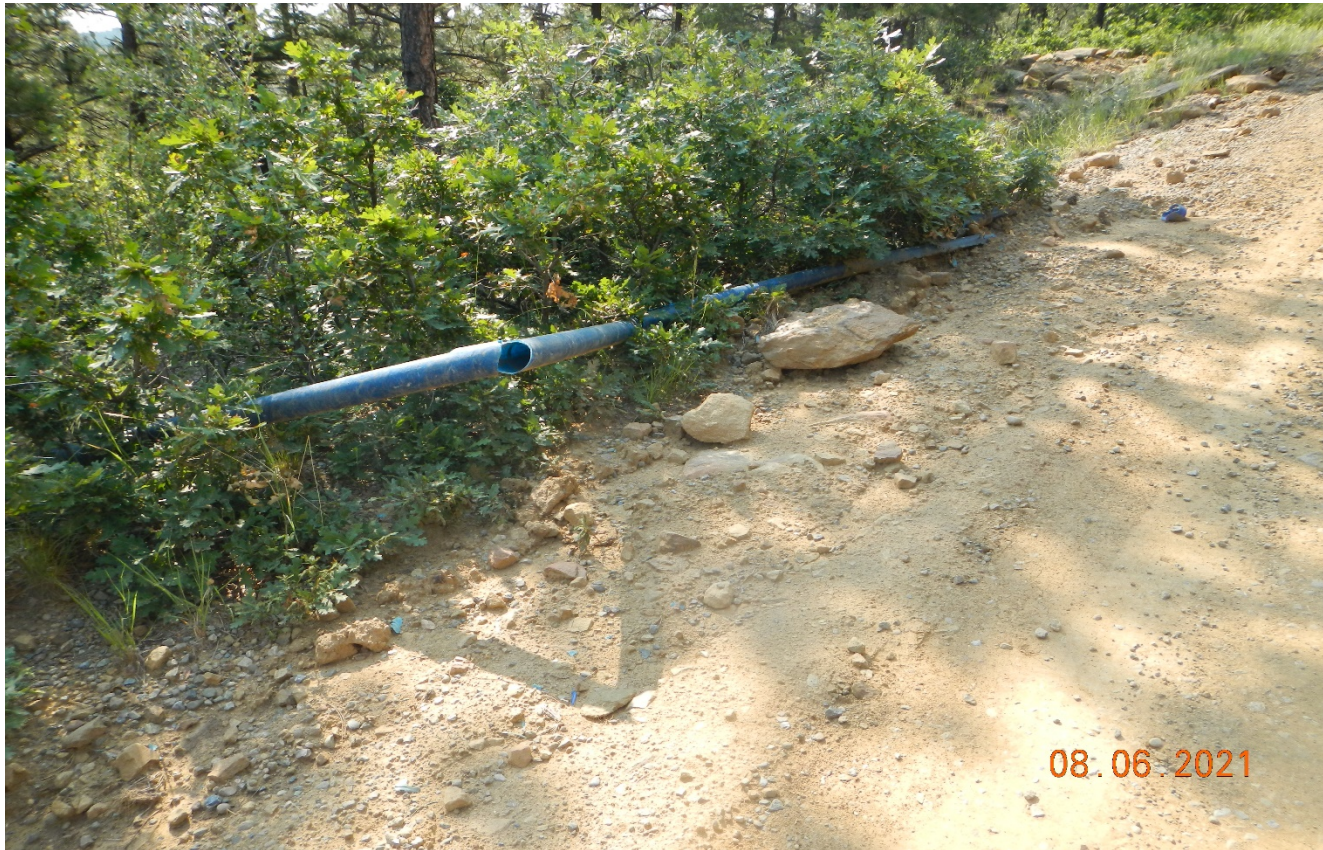
Photo 6. There is blue fiberglass pipe along area of the road that is broke apart and is trash. The pipe debris needs to be removed.
