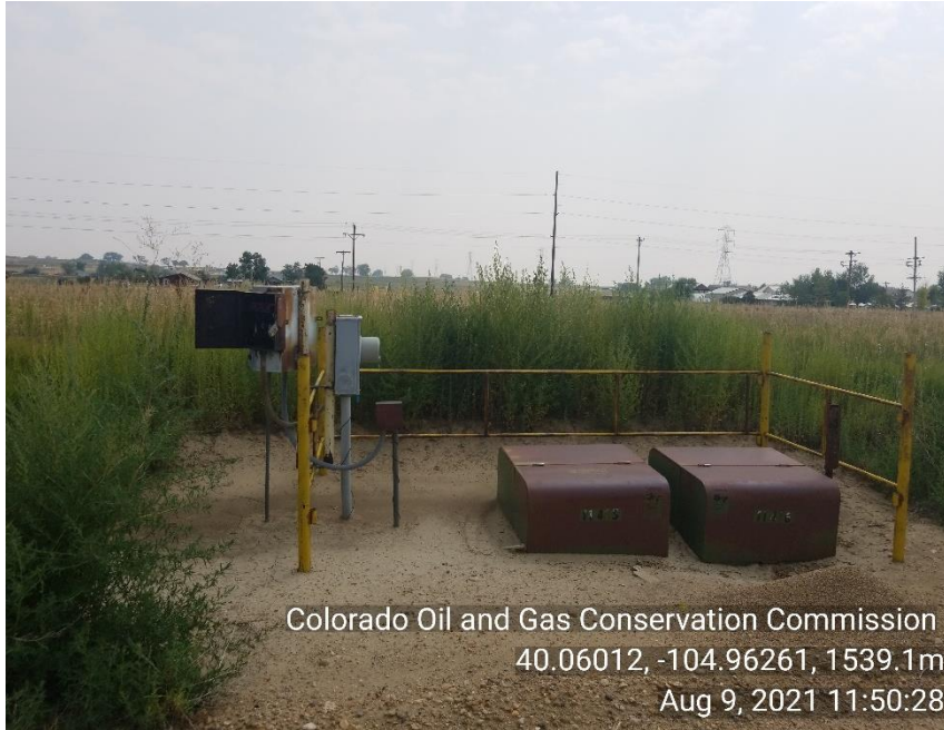
Photo 3 Electric panel. Meter is not on.
