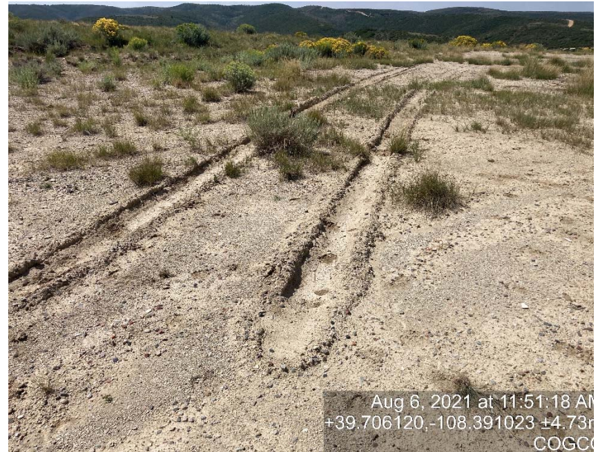
lack of stabilization/compaction
