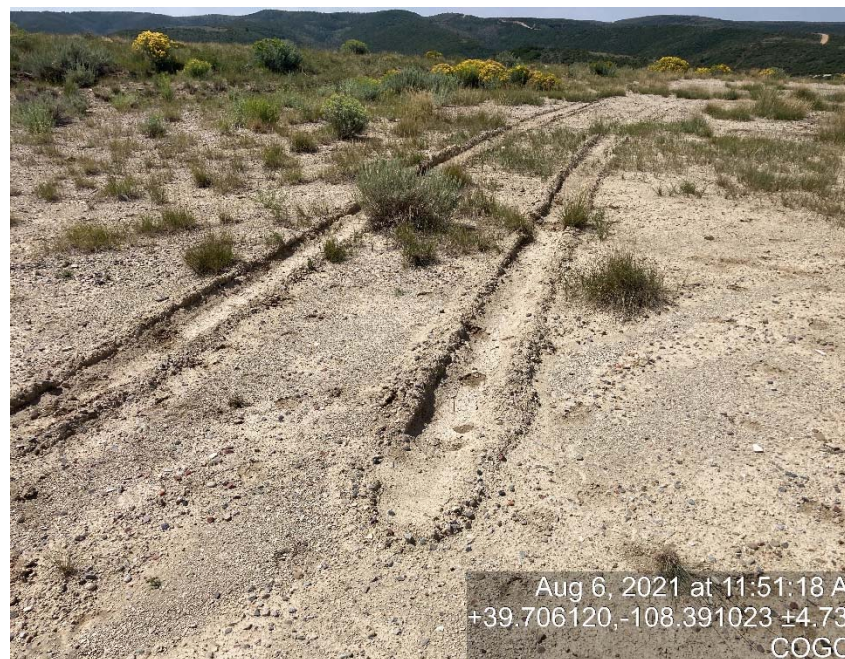
lack of stabilization/compaction
