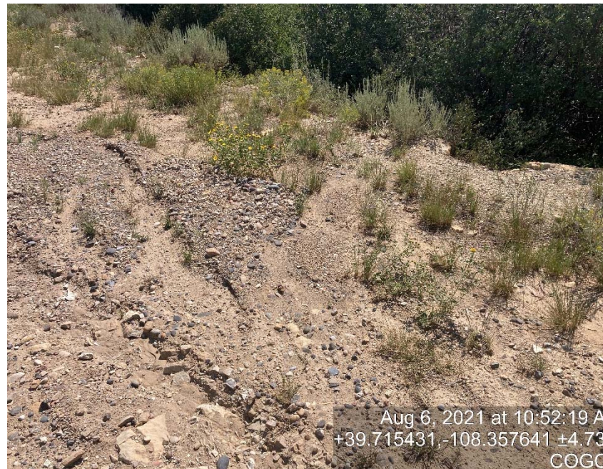
Access road erosion/lack of stabilization/compaction
