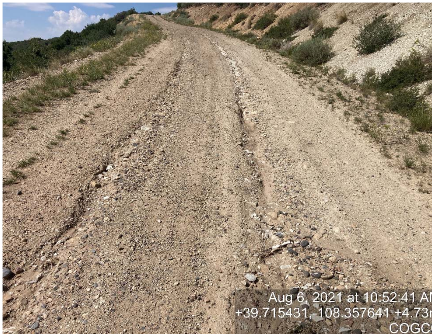
Access road erosion/lack of stabilization/compaction
