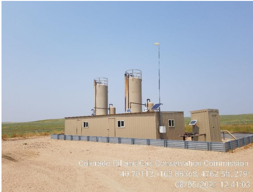
Photo 3 – Heater Treater and Gas Meter
