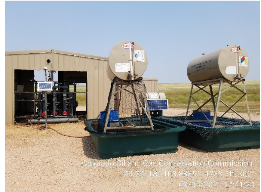
Photo 6 – Compressor – Wildlife Netting on Day Tanks
