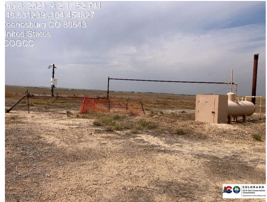
Pic 2 Gas meter run, separator.
