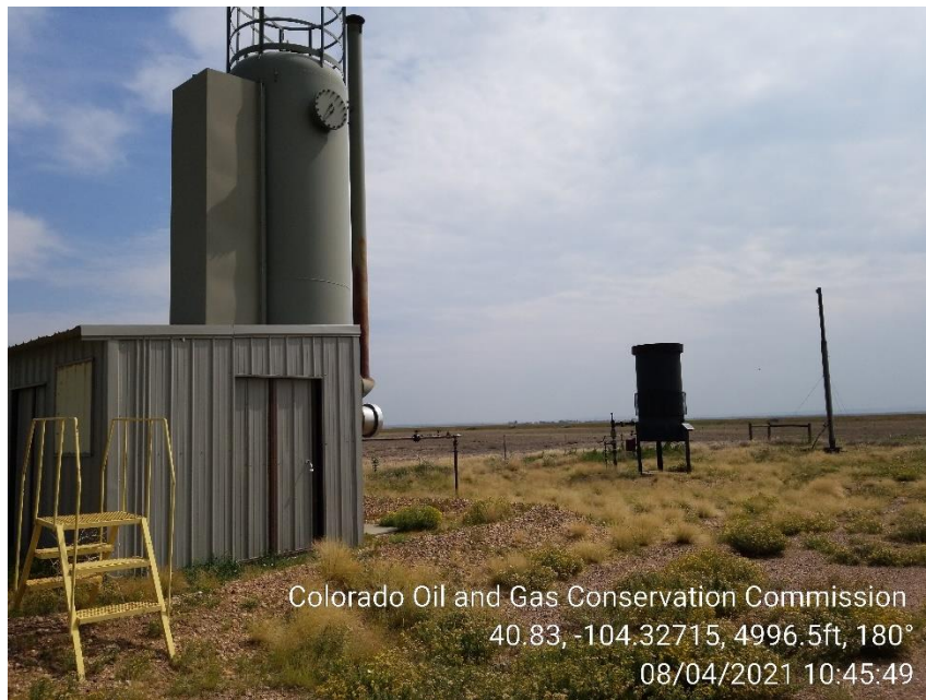
Photo 7 – Heater Treater, ECD and Flare
