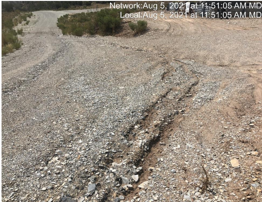
Photo #4721 Access road lacks stabilization.
