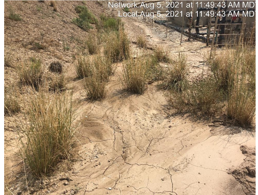
Photo #4716 Ditch is filled with sediment.
