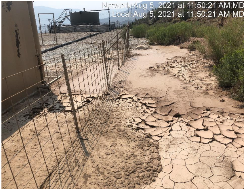
Photo #4719 Sediment is encroaching on production equipment.
