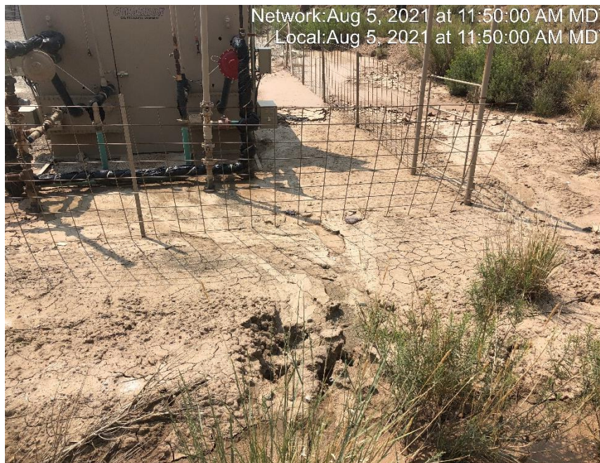
Photo #4717 Sediment is encroaching on production equipment.
