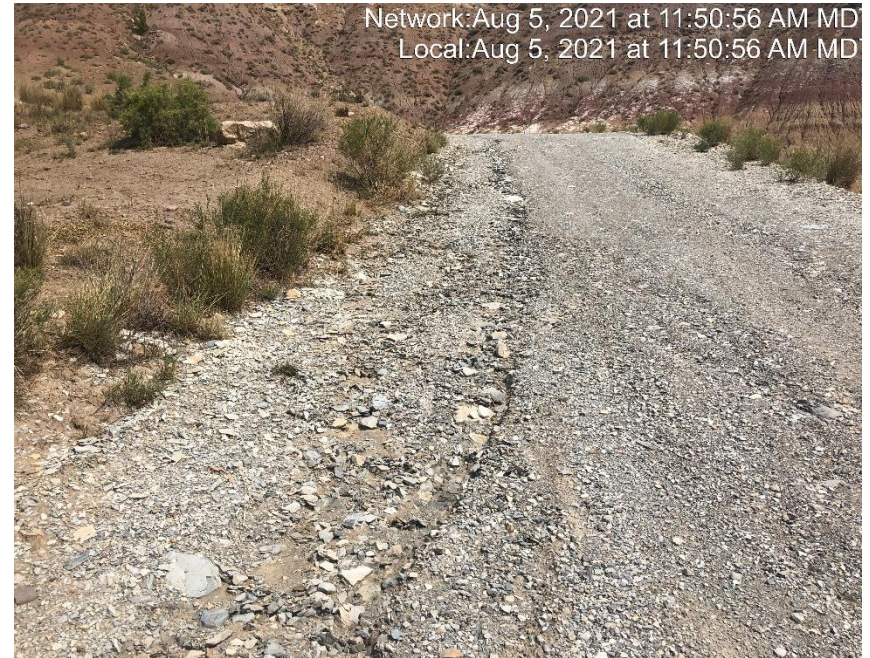
Photo #4720 Access road lacks stabilization.
