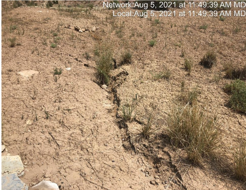
Photo #4715 Rill erosion occurring on cut slope.
