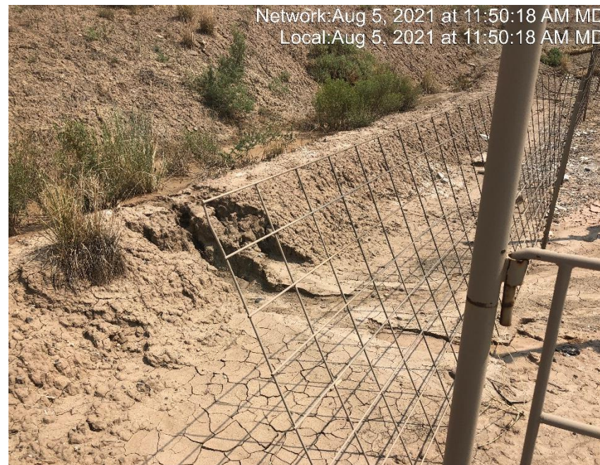
Photo #4718 Ditch is no longer controlling run on to location.
