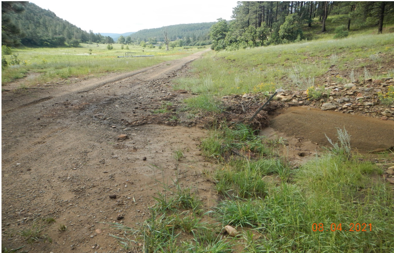
Photo 2. Facing back to the southeast at the culvert filled in with sediment.
