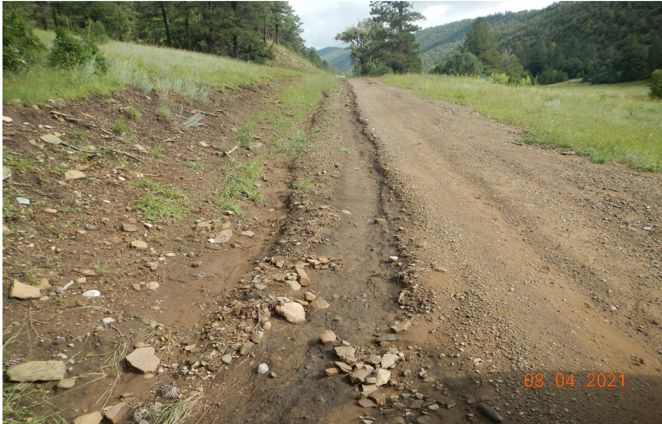
Photo 1. Facing northwest along the road traveling to the location. There A culvert further up is filled in with sediment causing erosion down the road in this area.
