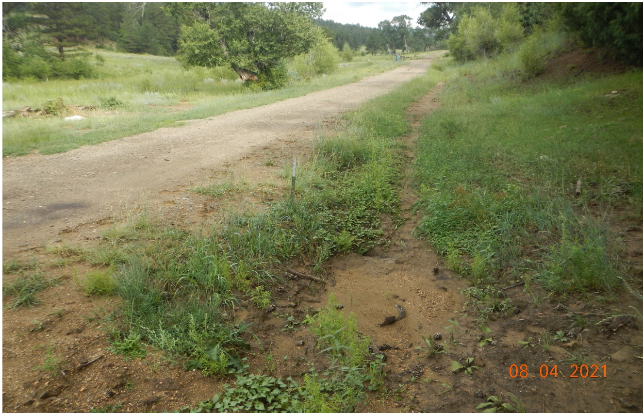
Photo 3. Further up the road in the canyon is another culvert filled in with sediment.
