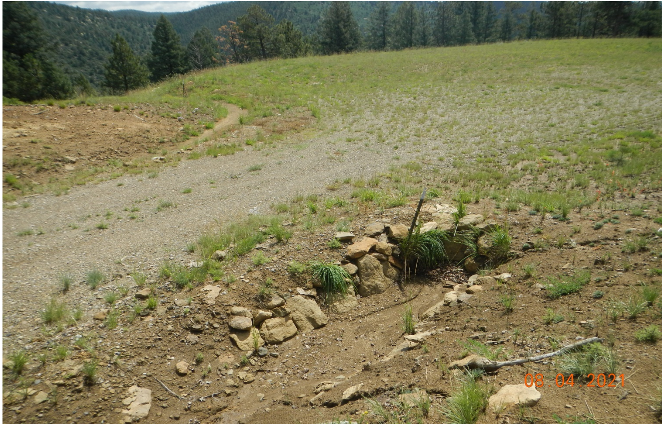
Photo 5. Facing southeast at the location. This culvert at the location has filled in with sediment.
