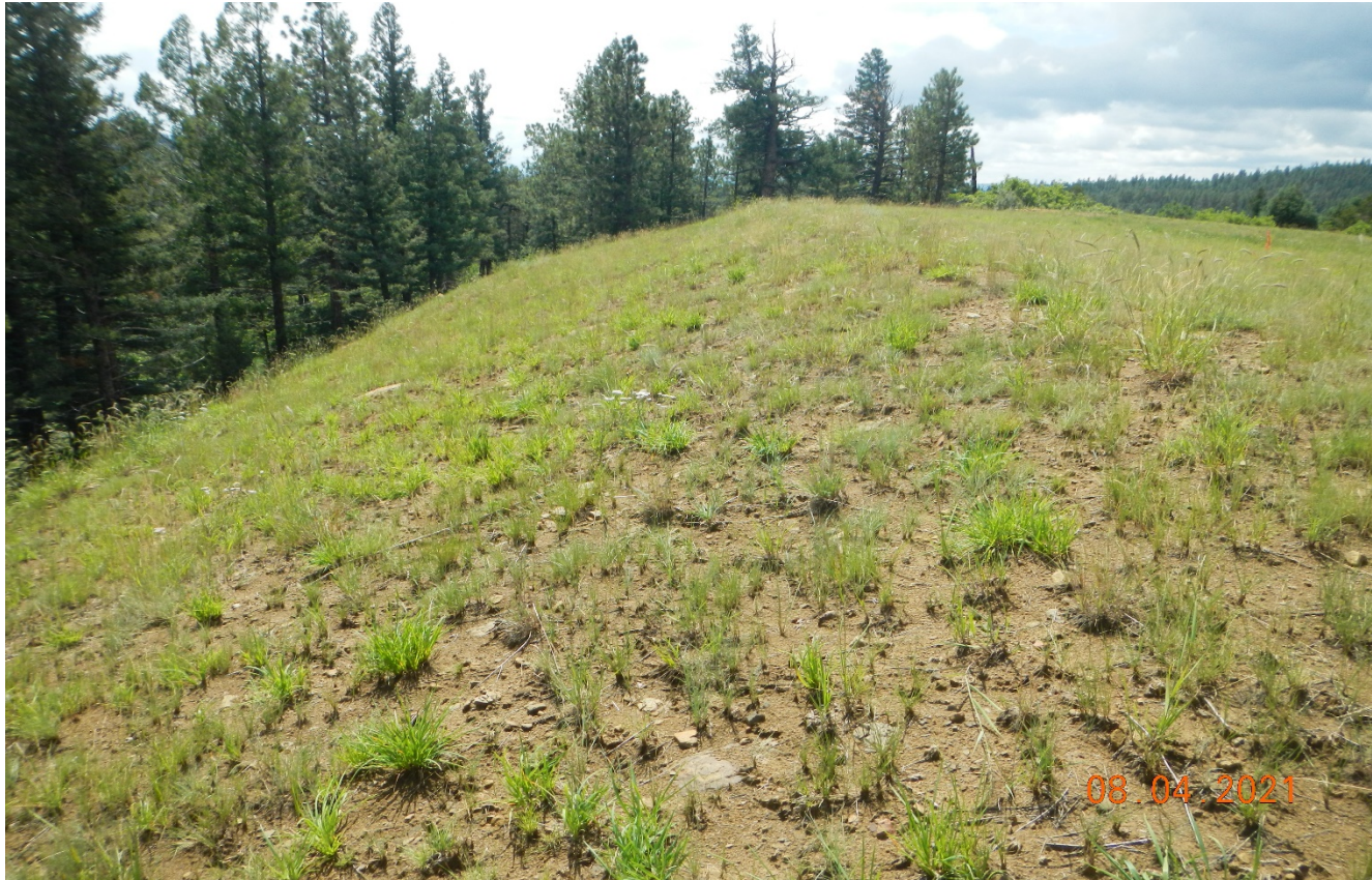
Photo 7. Facing southeast along the fill slope of the location. Perennial vegetation is well established along this area.
