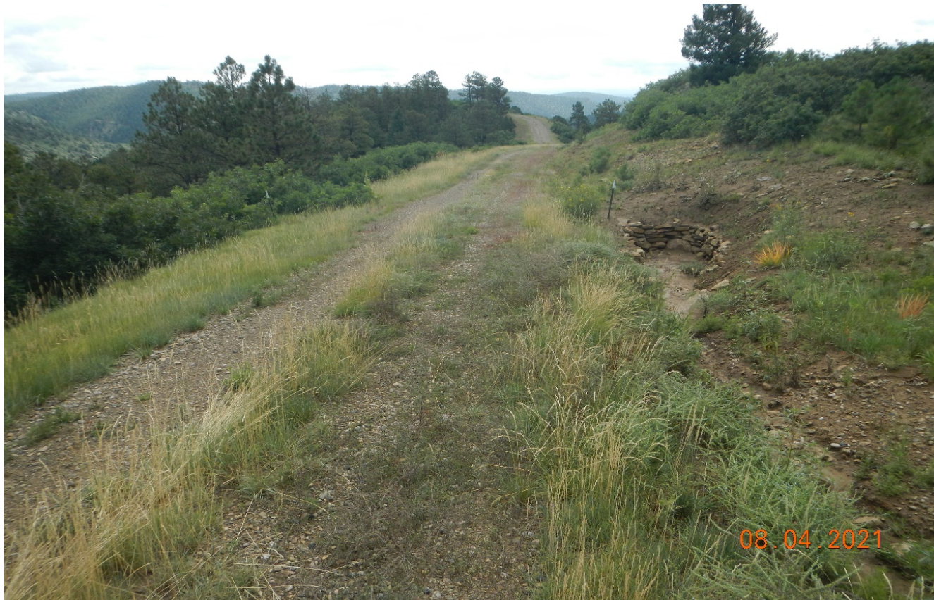
Photo 2. The access road is stabilized with gravel and vegetation. Culverts along the road are maintained.
