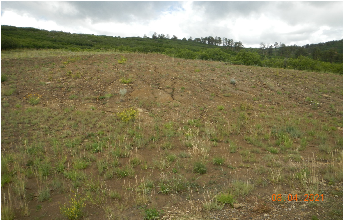
Photo 6. North side of the location facing west. There is signs of erosion along the slope. This area needs additional seeding to help establish vegetation.
