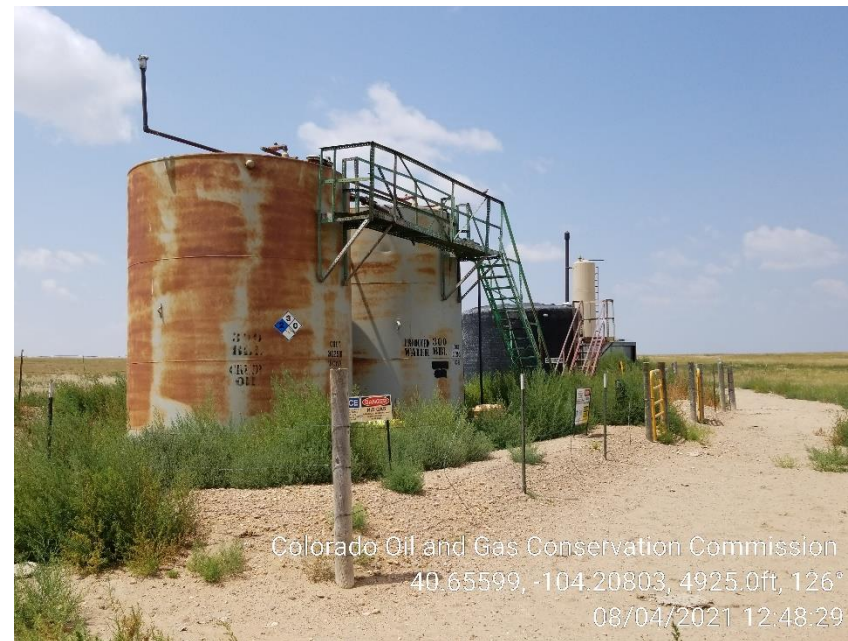
Photo 2 – Tank Battery
