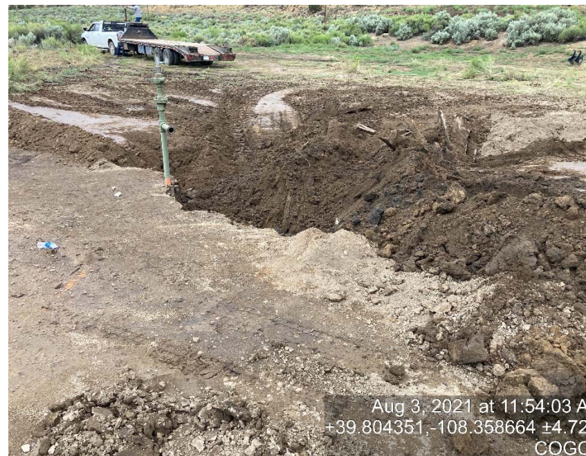
Well head location being filled in
