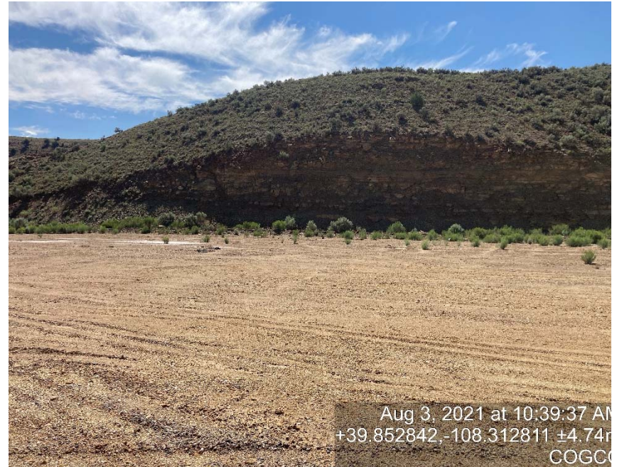
Cut slope not stabilized
