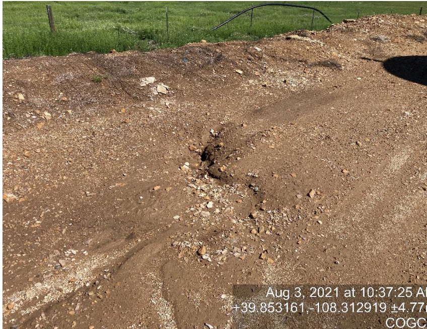
Lack of stabilization/erosion
