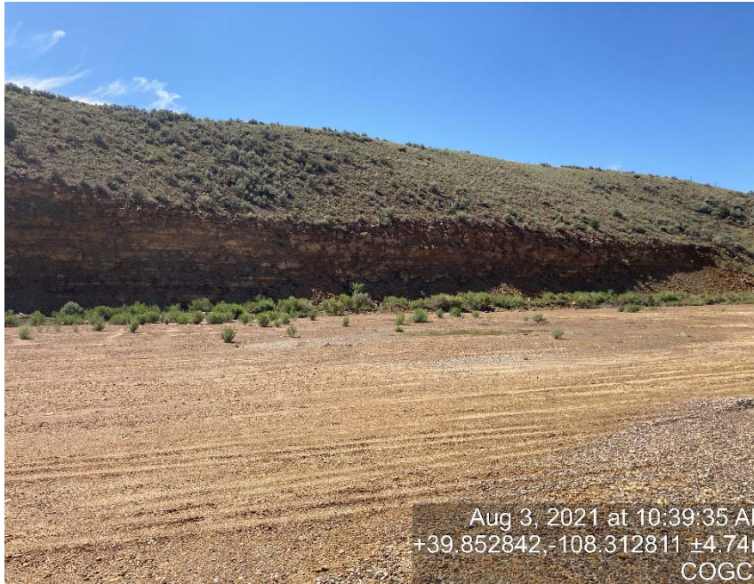
Cut slope not stabilized
