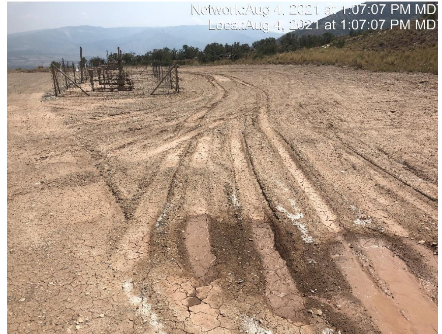
Photo #4696 Location lacks stabilization.
