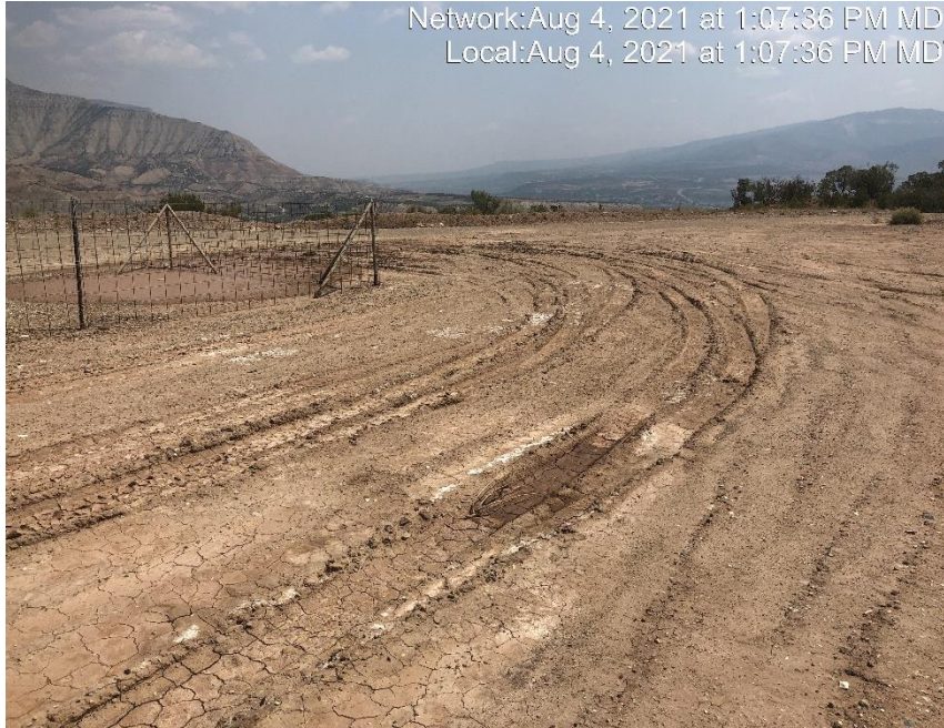
Photo #4698 Location lacks stabilization.
