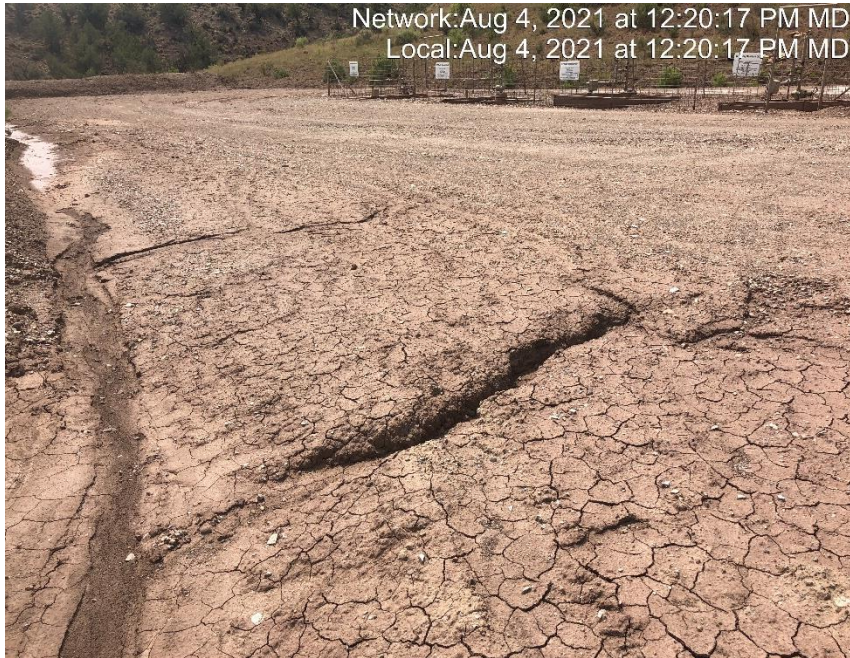
Photo #4691 Location lacks stabilization.
