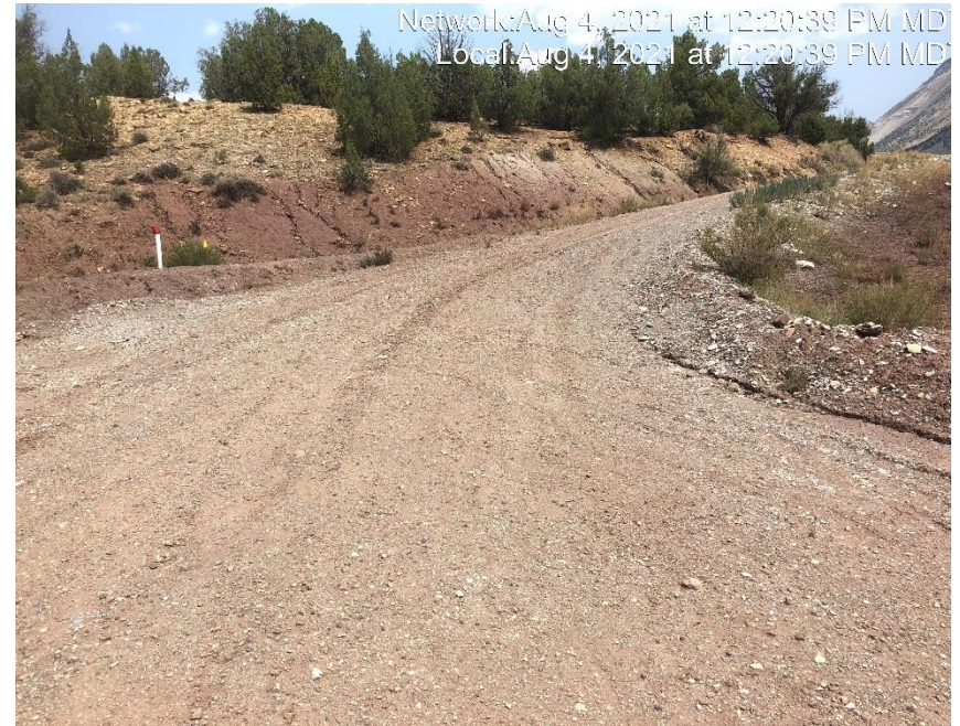
Photo #4692 No form of tracking BMP at entrance to location.
