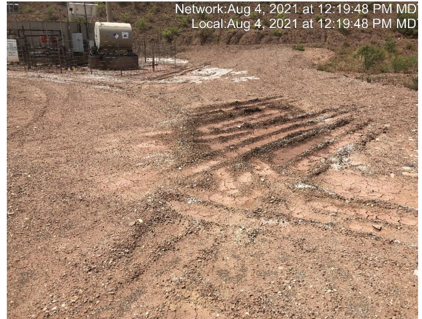
Photo #4690 Location lacks stabilization.
