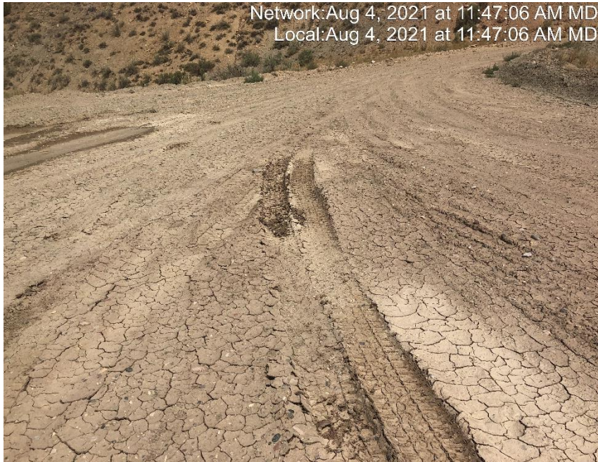
Photo #4686 No form of tracking BMP at entrance to location.
