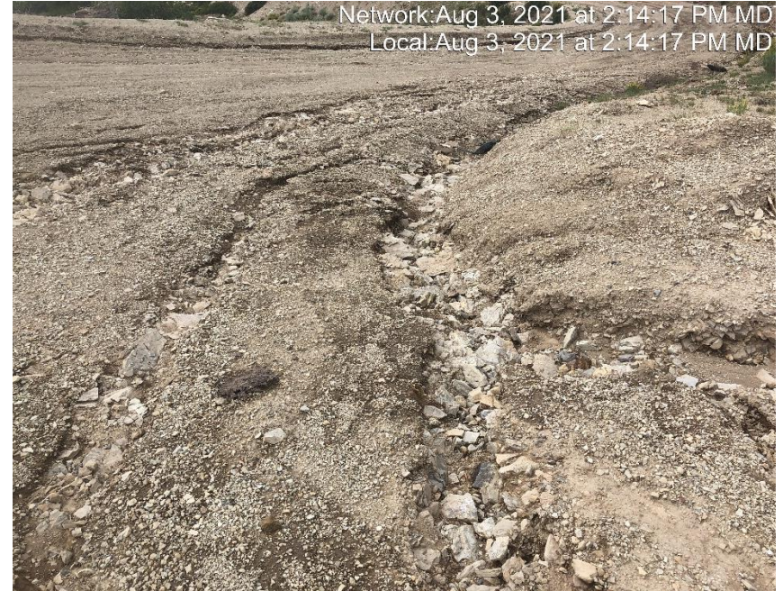
Photo #4681 Insufficient velocity check.
