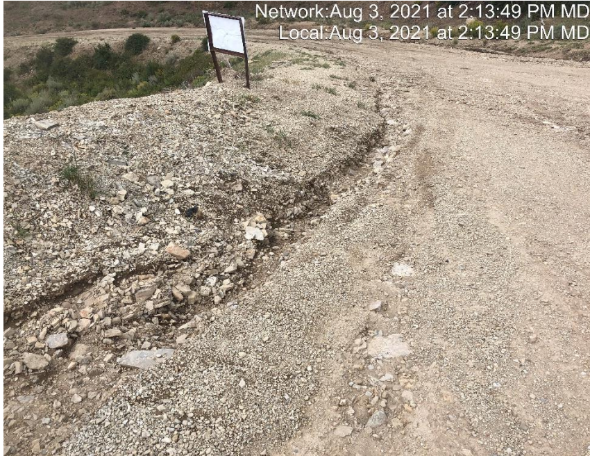
Photo #4678 Rill erosion occurring in ditch.
