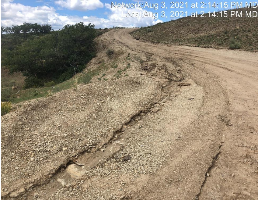
Photo #4680 Insufficient velocity checks.
