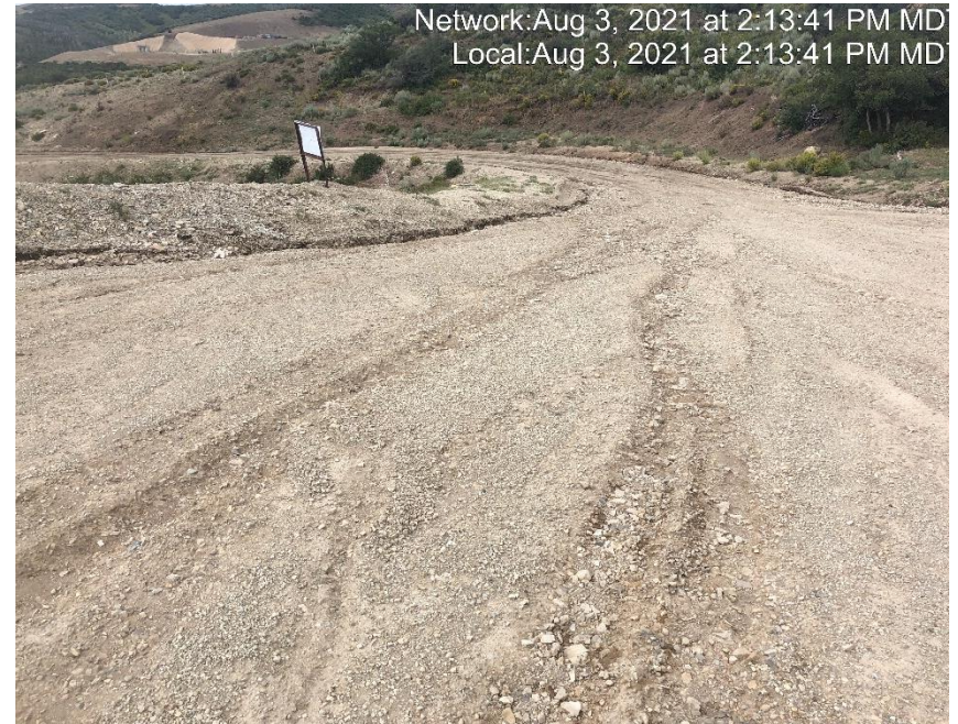
Photo #4677 Access road lacks stabilization.
