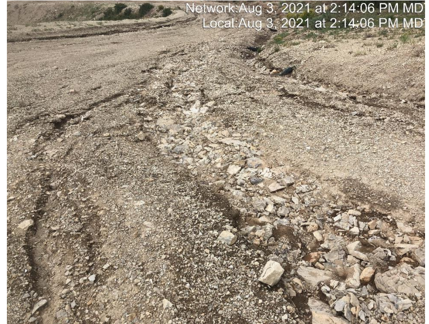
Photo #4679 Rill erosion occurring in ditch and access road.
