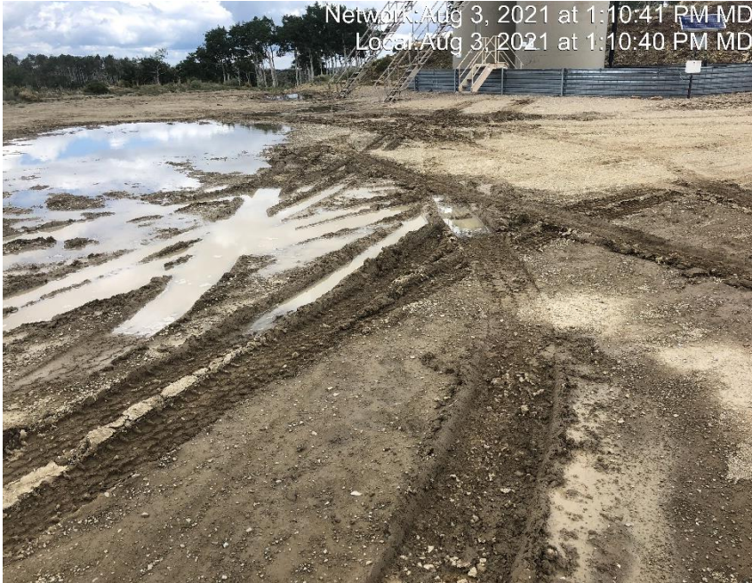
Photo #4665 Location lacks stabilization.
