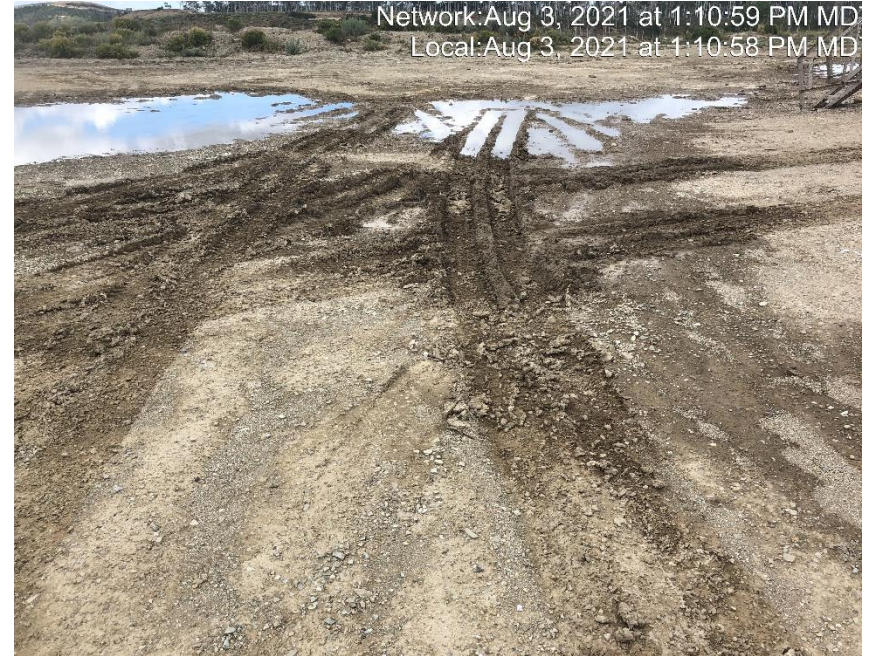
Photo #4666 Location lacks stabilization.
