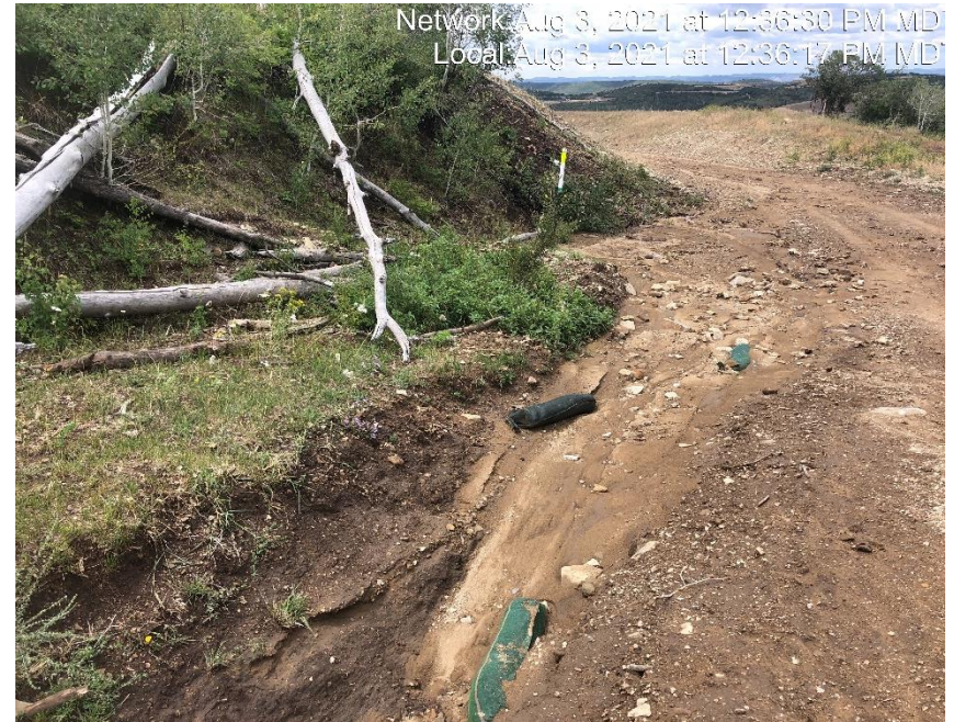
Photo #4659 Sediment has been transported onto access road.
