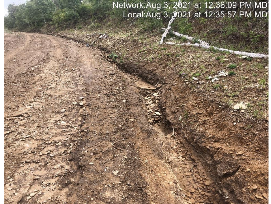
Photo #4657 Insufficient velocity checks in ditch.
