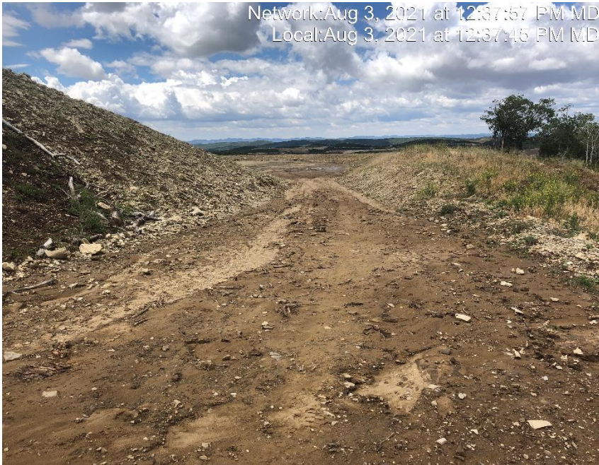
Photo #4662 Sediment has been transported down access road.
