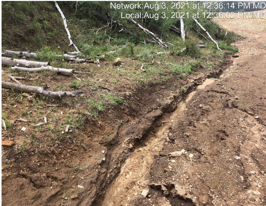
Photo #4658 Gully erosion occurring in ditch.
