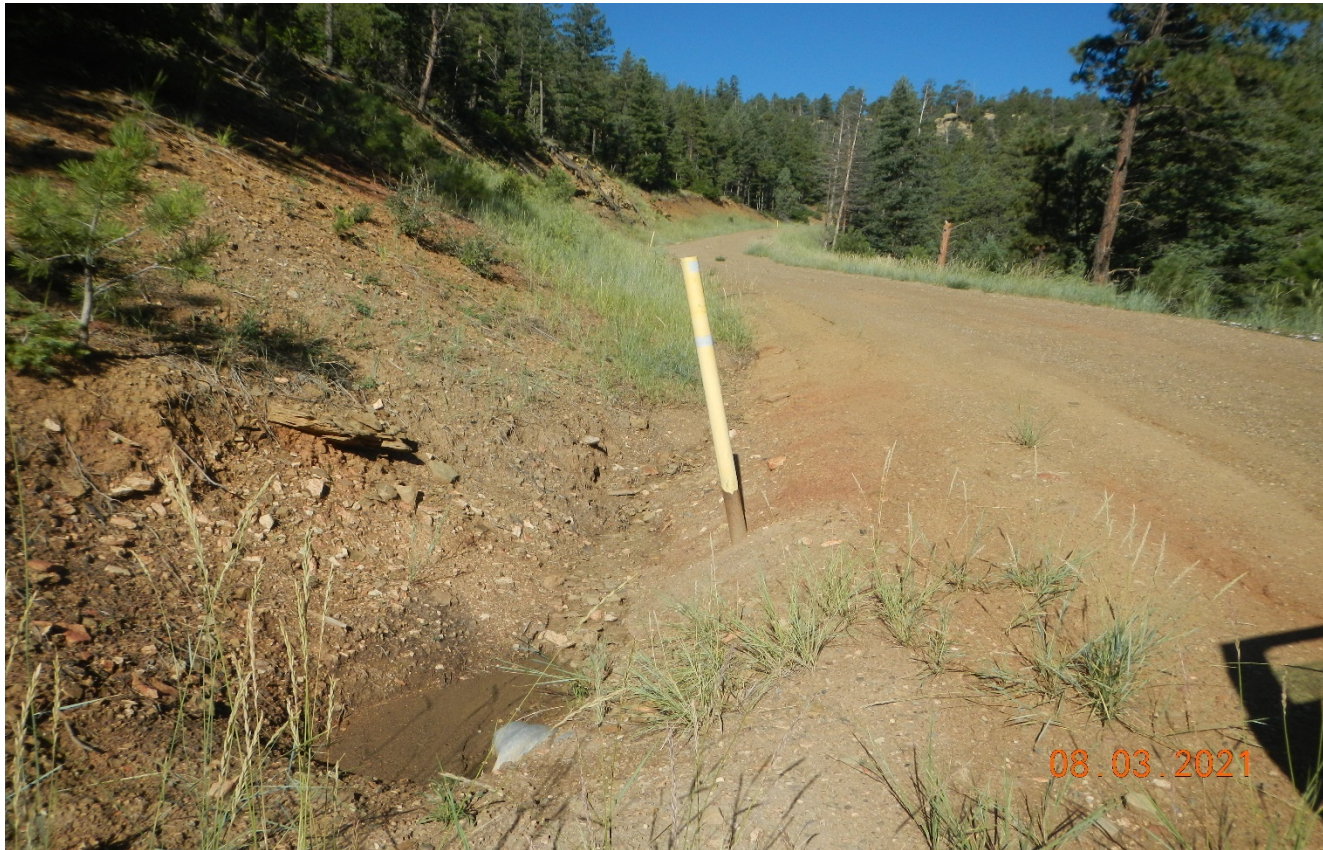
Photo 2. The culvert along the road has been repaired. There is some sediment beginning to accumulate which should be cleaned before it fills in.
