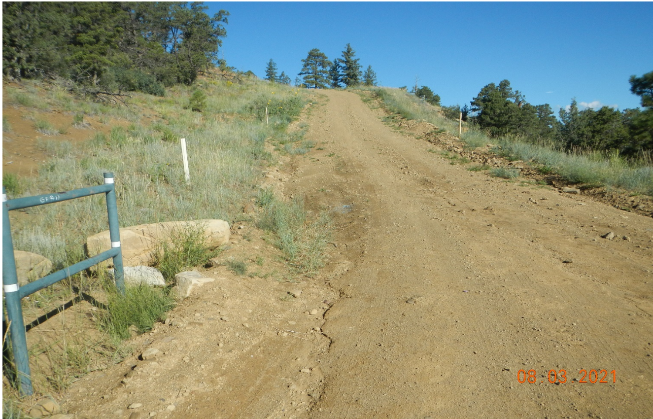
Photo 4. Facing northwest toward the access road that continues past the location. The road has been graded and culverts are maintained.
