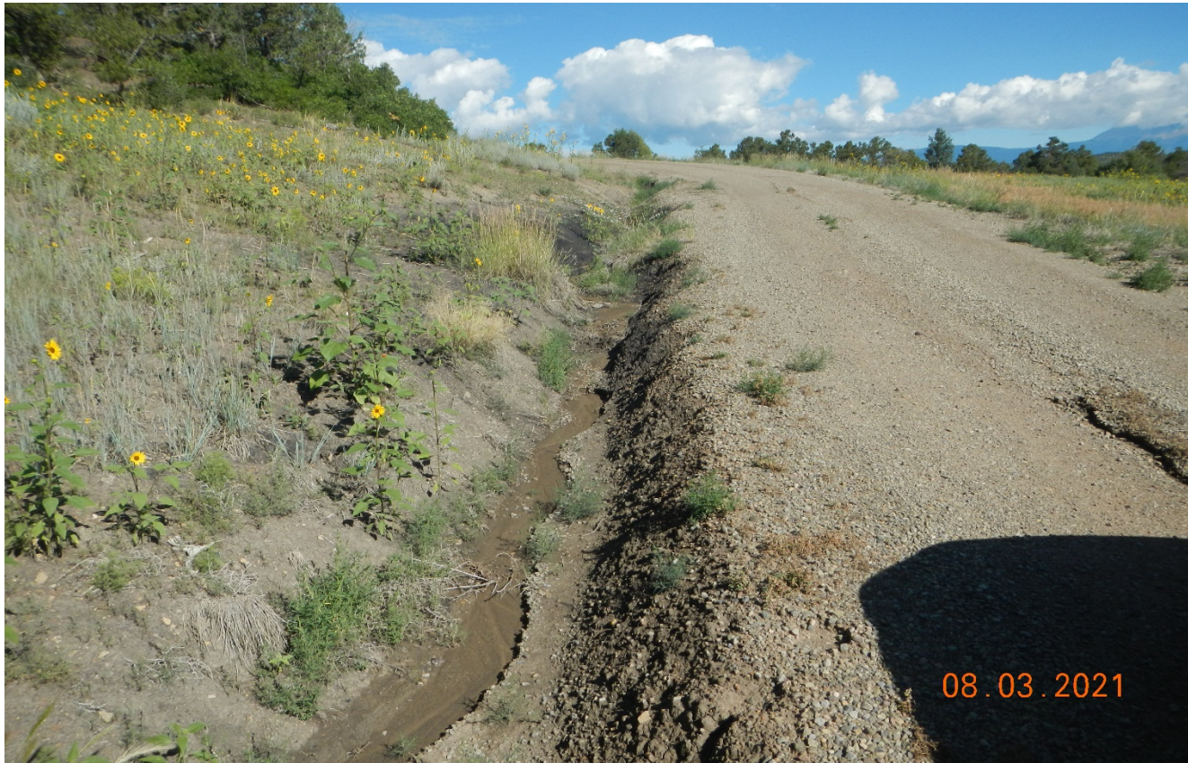
Photo 1. Facing northeast along the main access road. There is erosion along the side of the road which needs BMP's to prevent further erosion.
