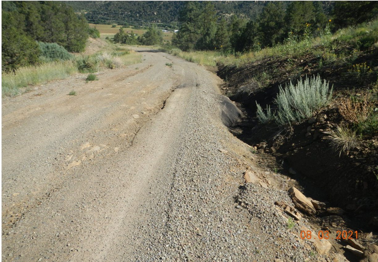
Photo 3. Facing back down the access road. There is erosion along the side of the road which needs BMP's to prevent further erosion.
