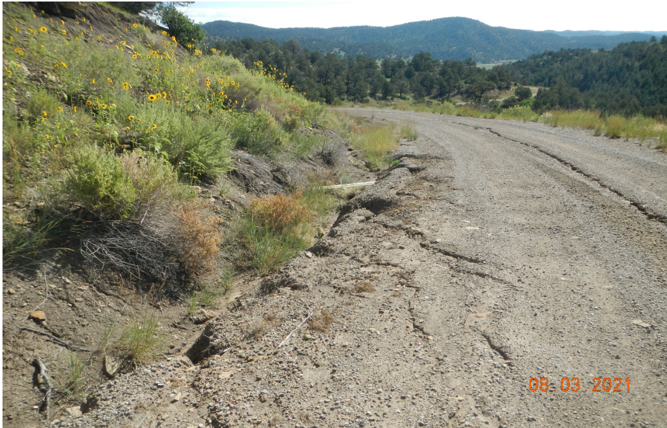
Photo 4. Facing back down the access road. There is erosion along the side of the road which needs BMP's to prevent further erosion.
