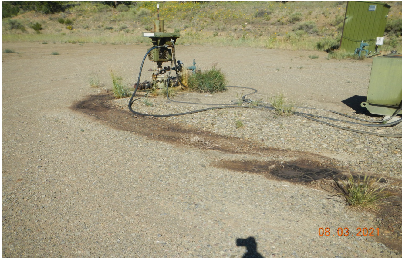
Photo 6. There is a dripping water leak at the wellhead which is shown by the staining on the surface.
