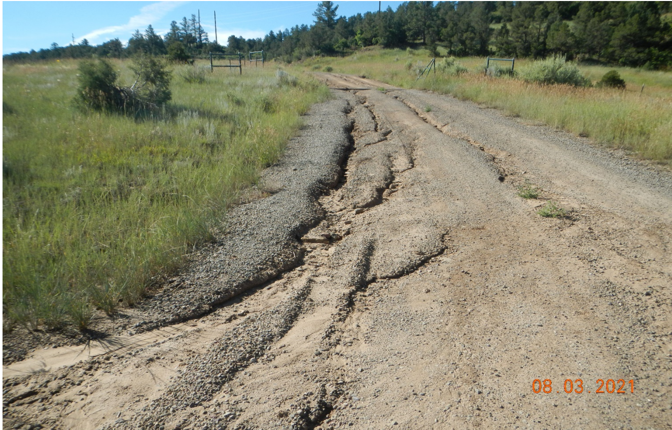
Photo 1. Facing southeast along the main access road. The erosion along the road needs to be repaired.
