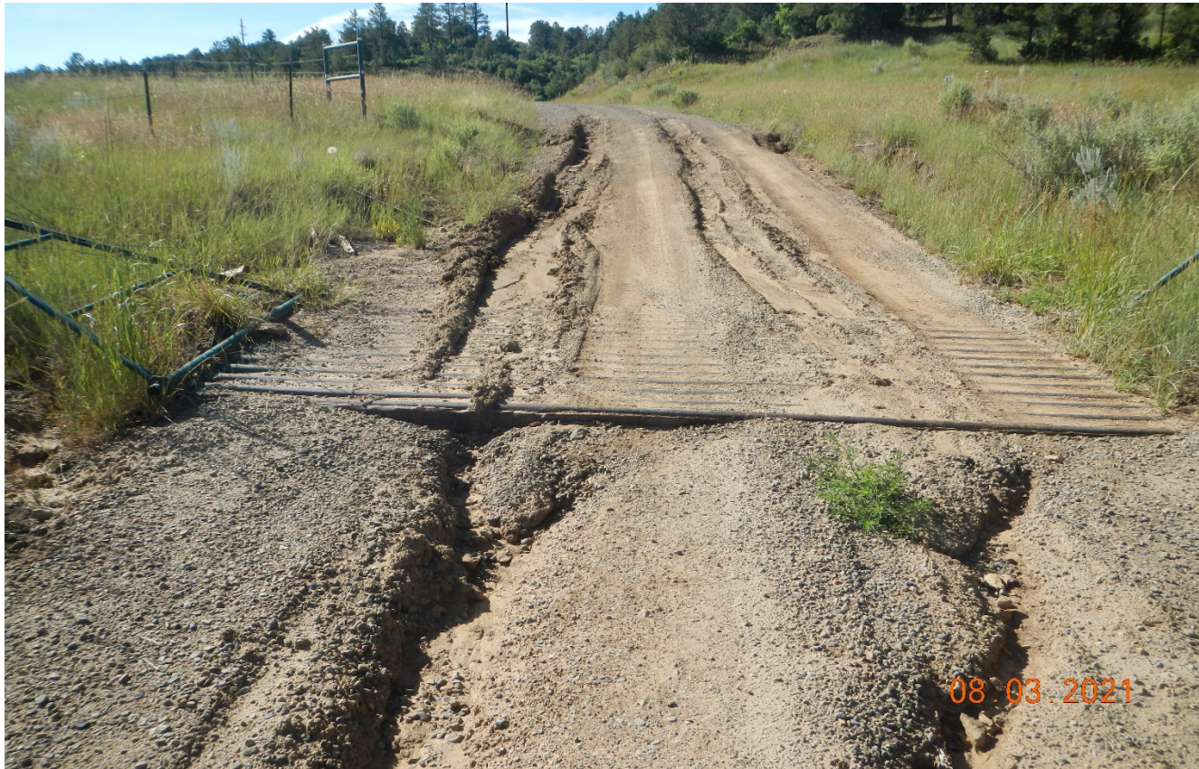
Photo 2. The cattle guard is filled in with sediment and needs to be repaired.
