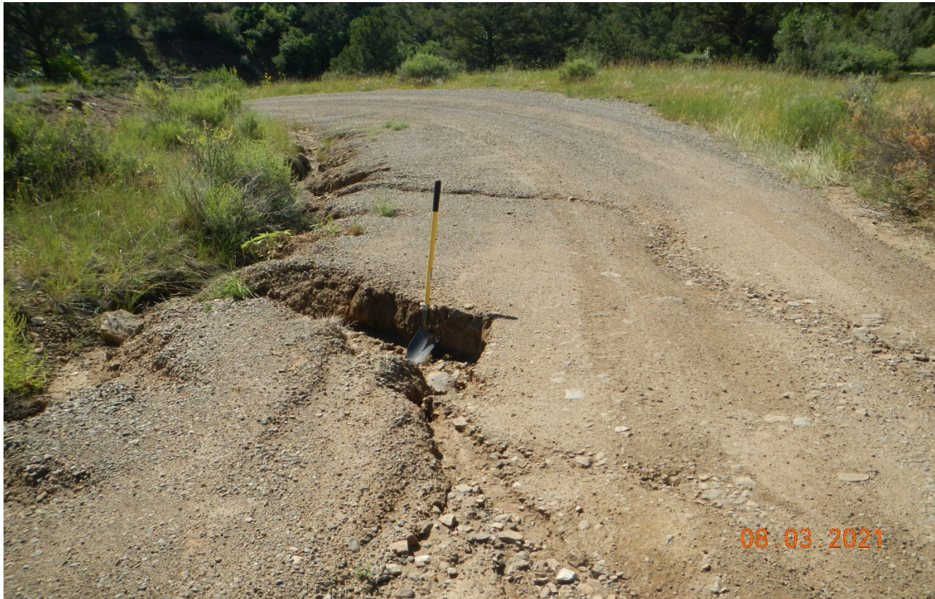
Photo 1. There is erosion along the access road near the location. Areas of erosion need to be repaired and stabilized.
