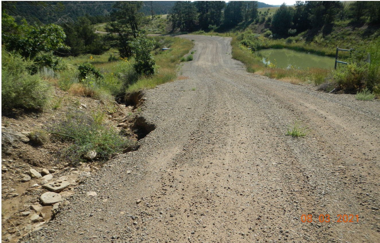
Photo 2. The erosion continues off the side of the road from previous photo. this area needs to be stabilized.
