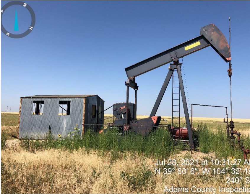
Photo #3 Pump jack.
