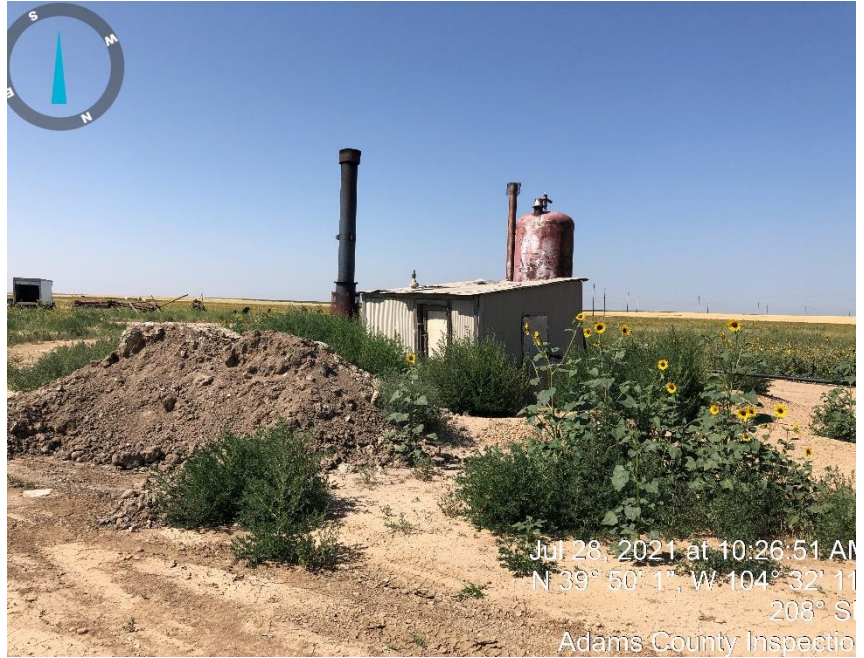
Photo #4 weeds and dirt pile on east side of separator.
