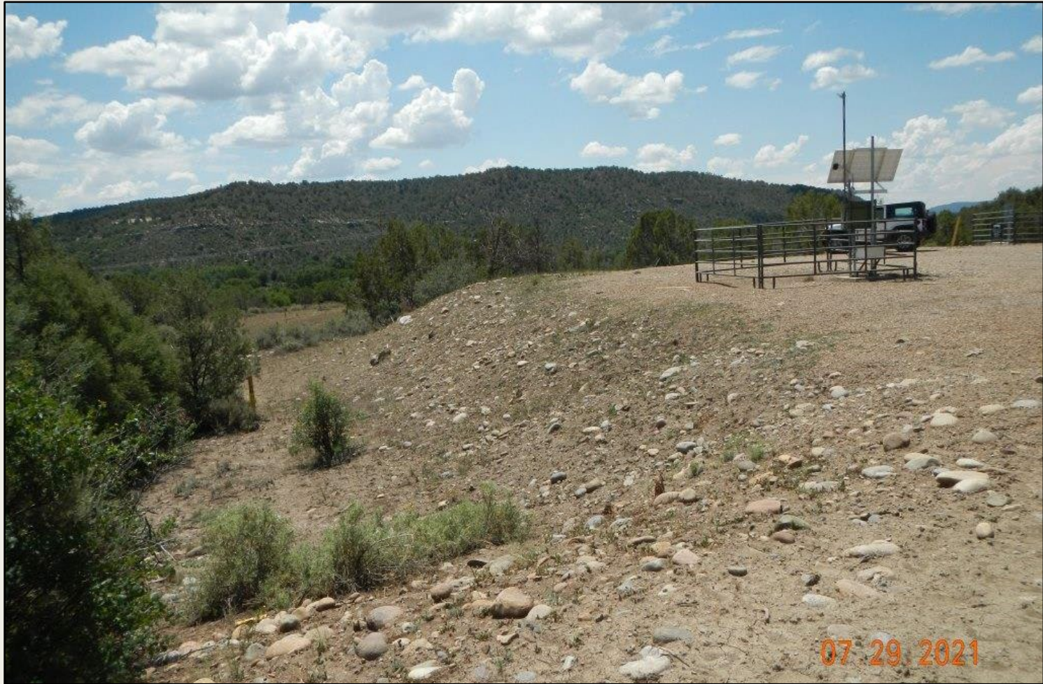
Photo 3. View of the southern project area from the southeastern corner facing southward. Vegetation here is grazed and sparse. Stormwater BMPs need to be installed and maintained until slope is stabilized.
