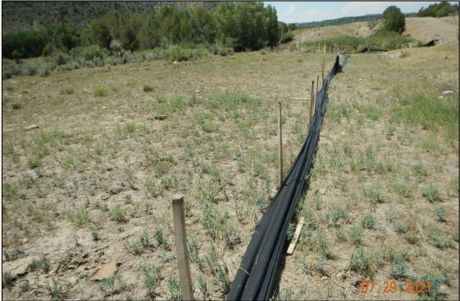
Photo 4. View of silt fence along the flowline right of way that is fallen, and no longer functioning.
