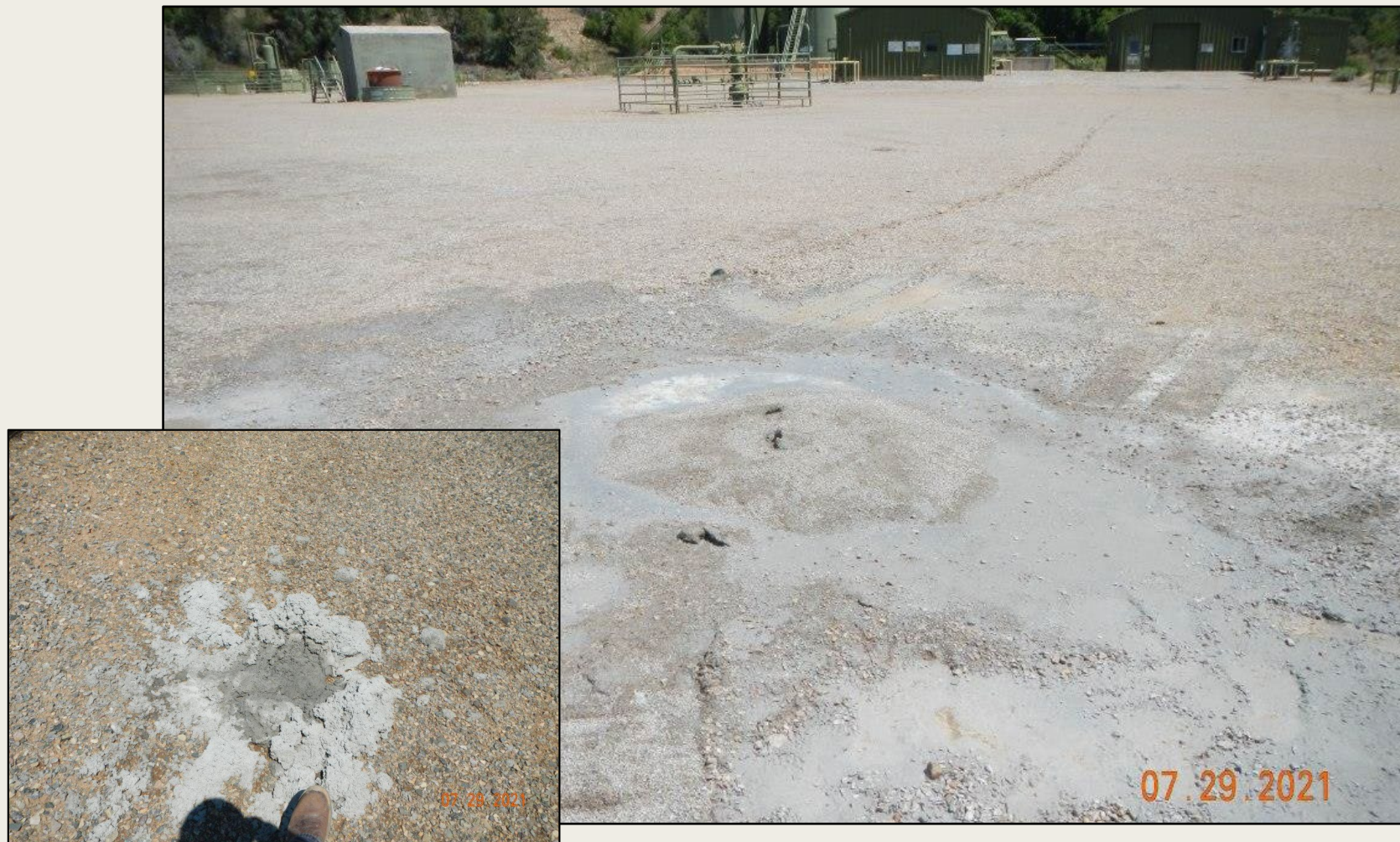
Photo 4. View of cement washout and debris in the southwestern well pad and in the southeastern well pad (inset). Needs to be removed and properly disposed of.
