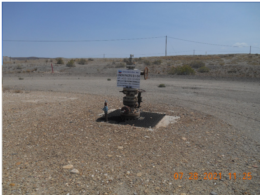
Injection wellhead. Temporarily Abandoned
