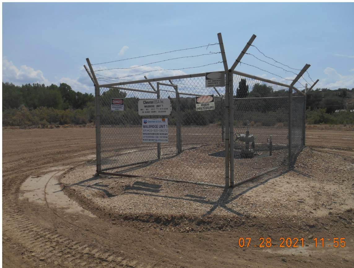
Injection wellhead – Temporarily abandoned
