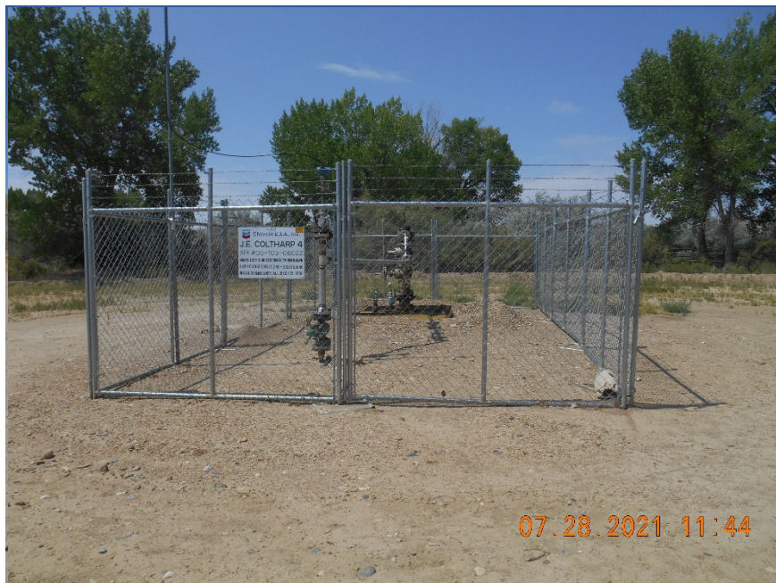
Injection wellhead. Temporarily Abandoned
