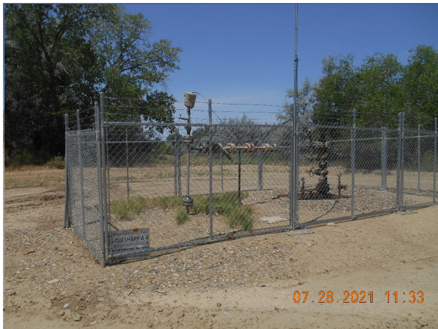
Injection wellhead. Temporarily Abandoned
