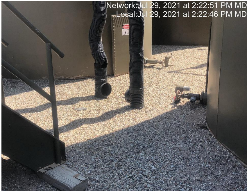
Photo #4624 Multiple flow line heating insulation open ended and not capped.
